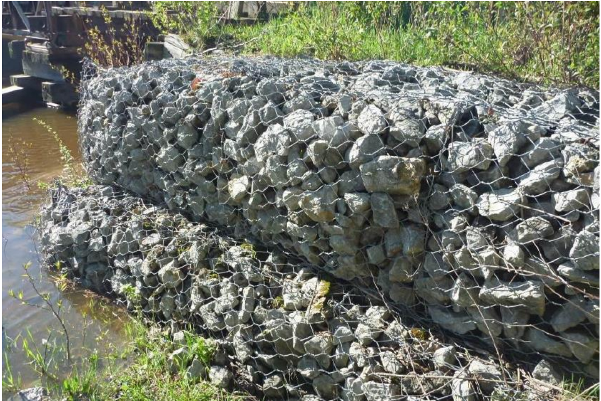
Photograph 5 –West Gabion Basket at West Abutment
