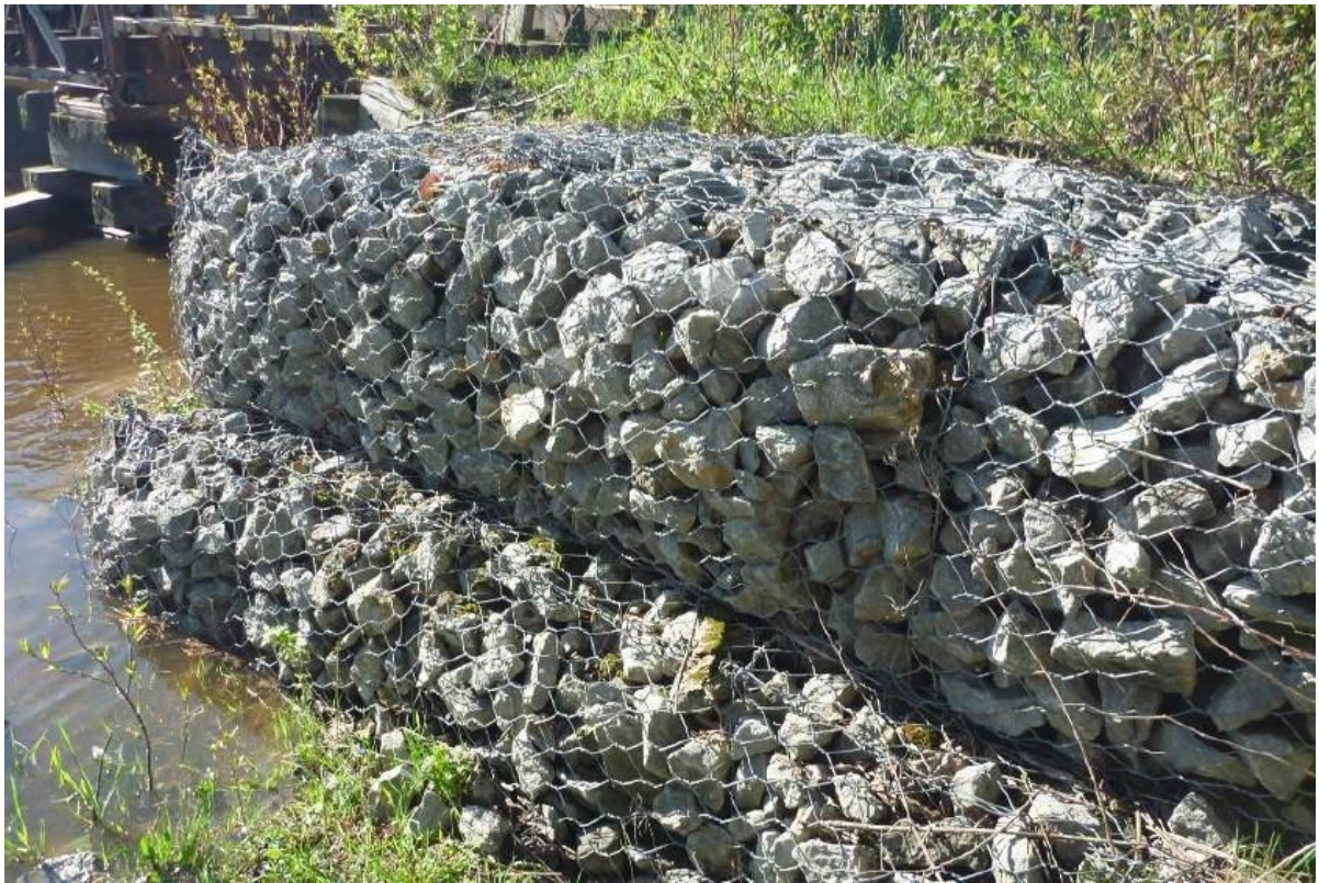
Photograph 5 –West Gabion Basket at West Abutment
