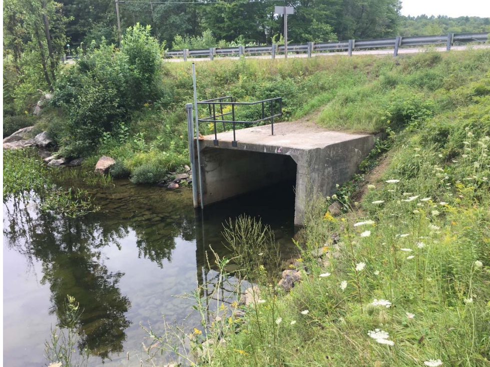
Photo 5. Outlet with water level measuring instrument (2017/08/17)
