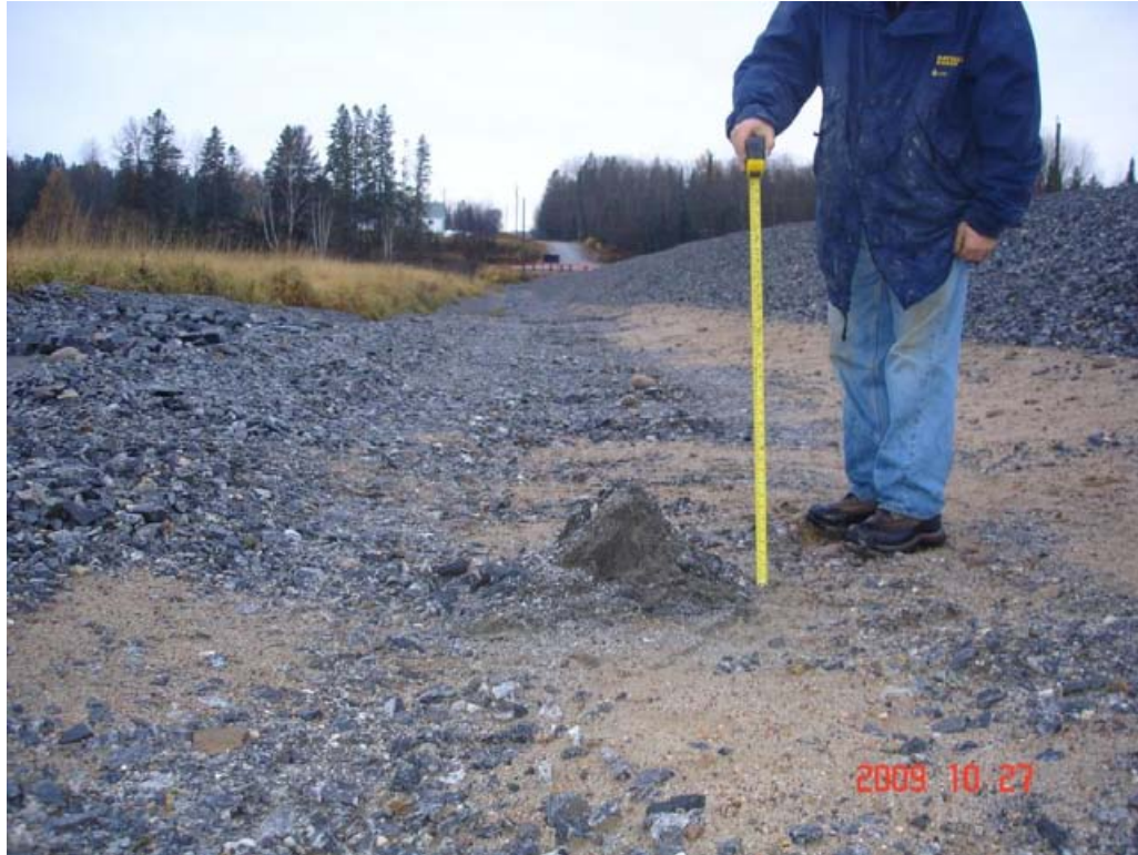
Figure E7 – Sand boil on south SSM slope (looking west)
