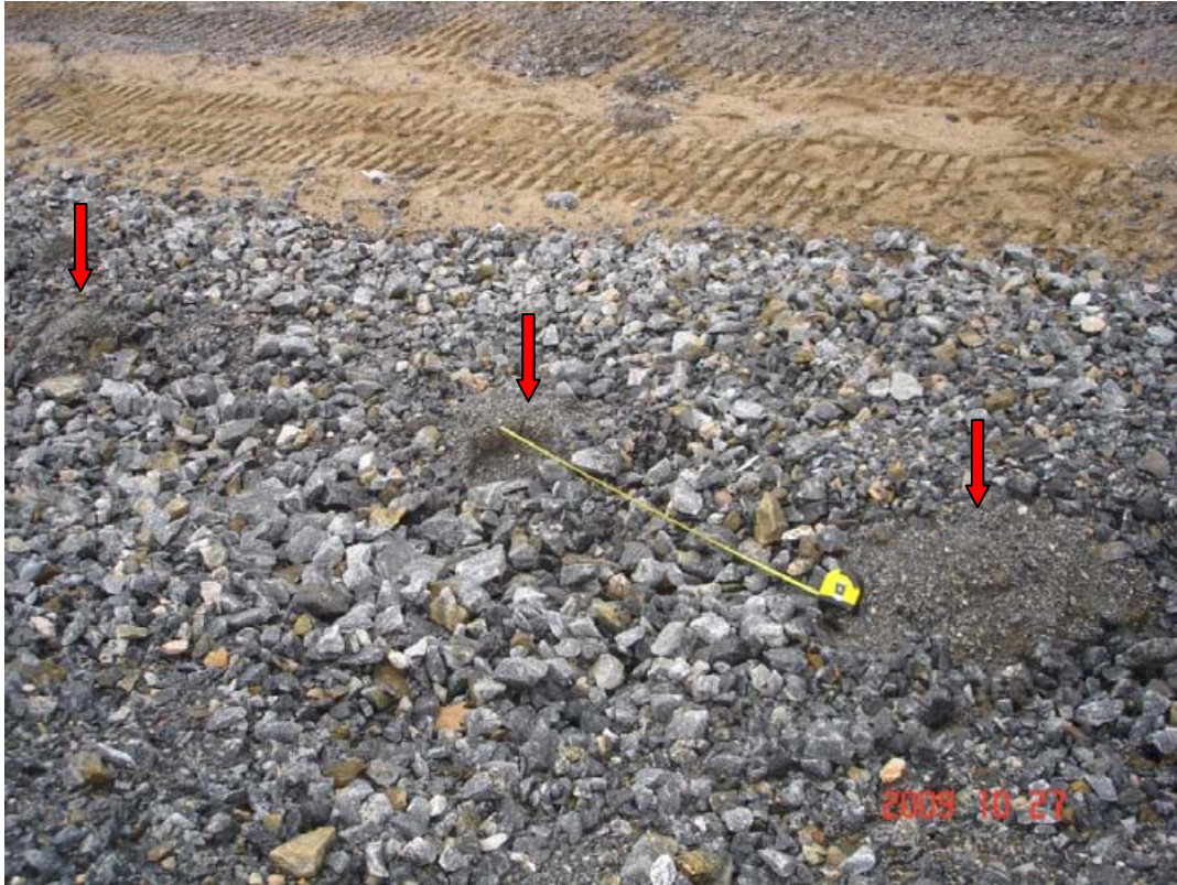
Figure E9 – Sand boils on south Granular B Type 2 Surcharge slope
