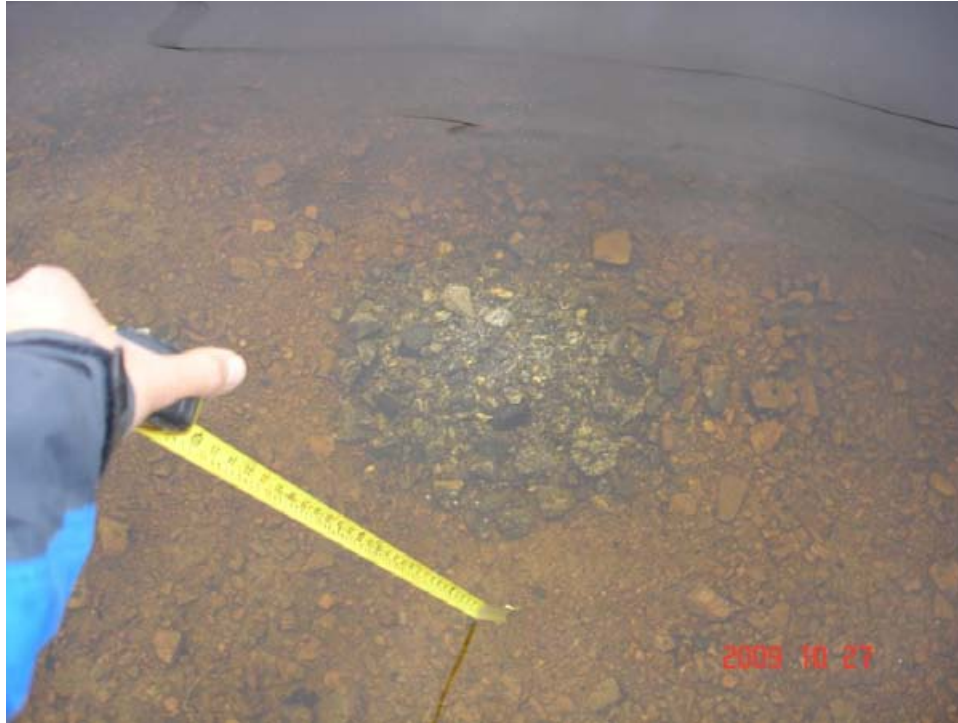
Figure E11 – Sand boil at the top of backfill in the north ditch
