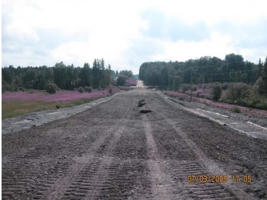
Figure E1 – Black Creek Road Embankment Instability on July 3, 2009 (looking west)
