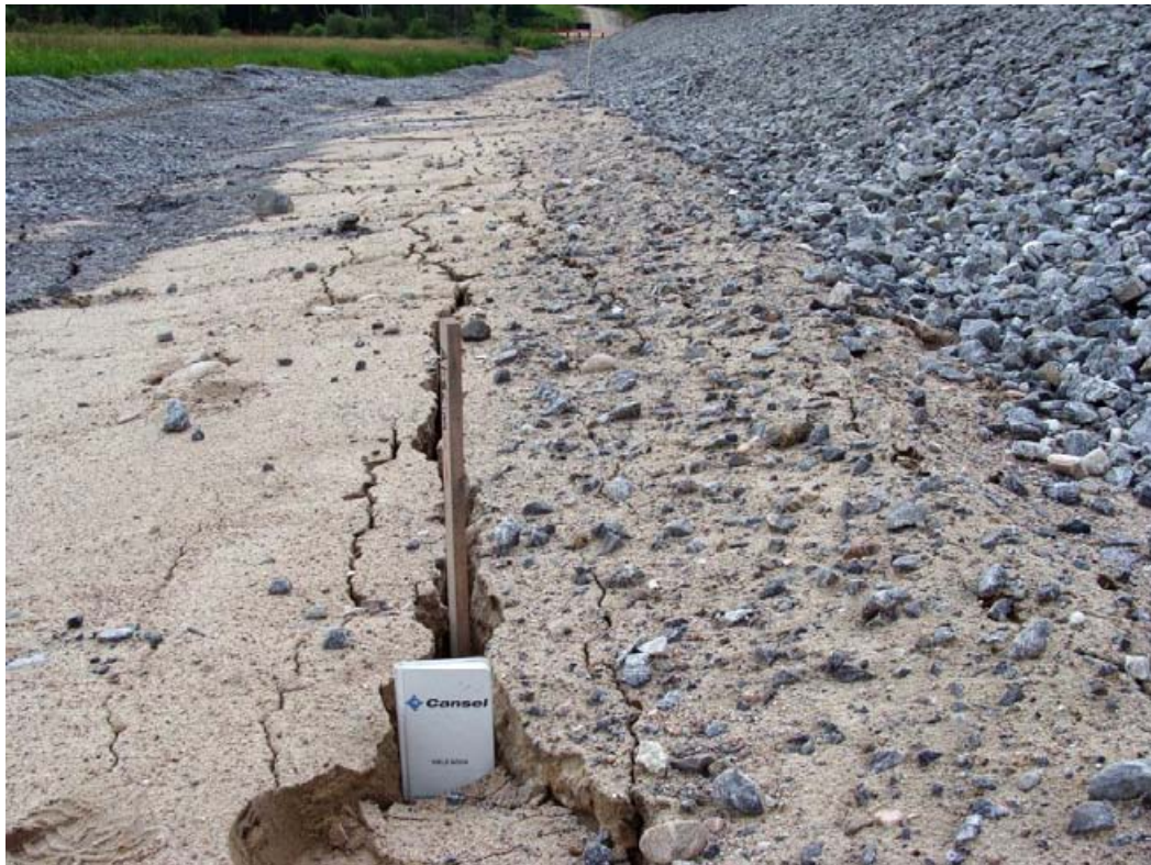
Figure E4 – Tension Cracks on the south SSM slope (looking west)
