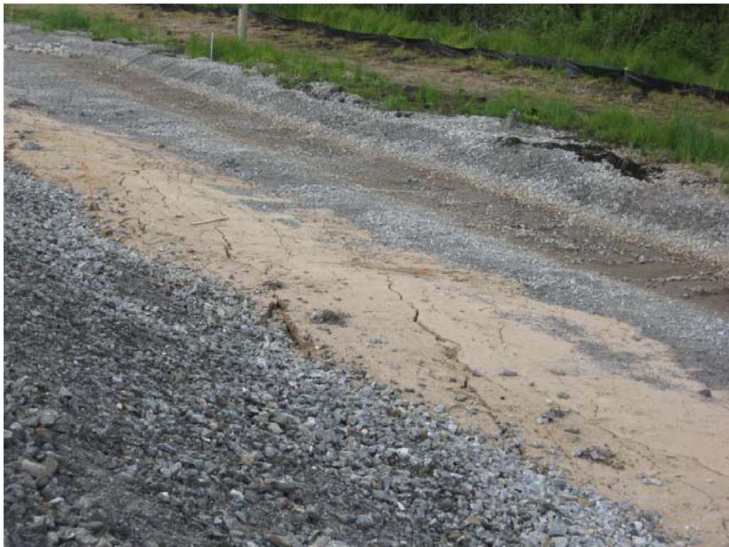
Figure E6 – north toe bulge (looking north west)
