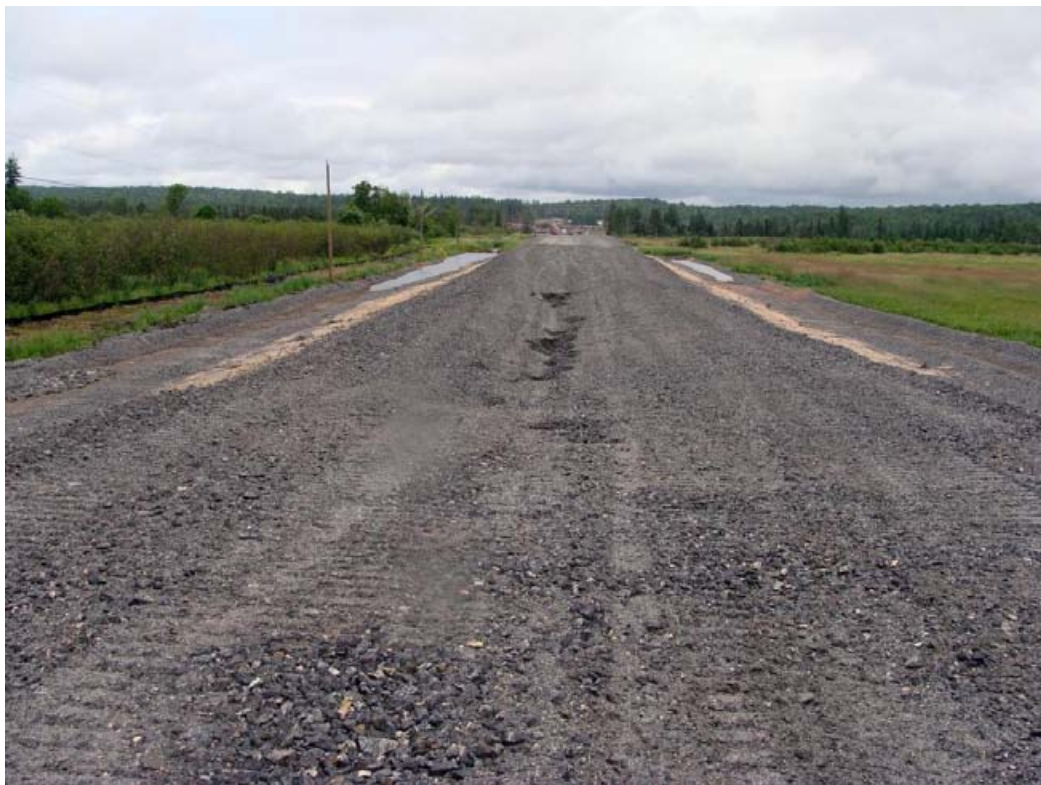
Figure E2 – Black Creek Road Embankment Instability (looking east)
