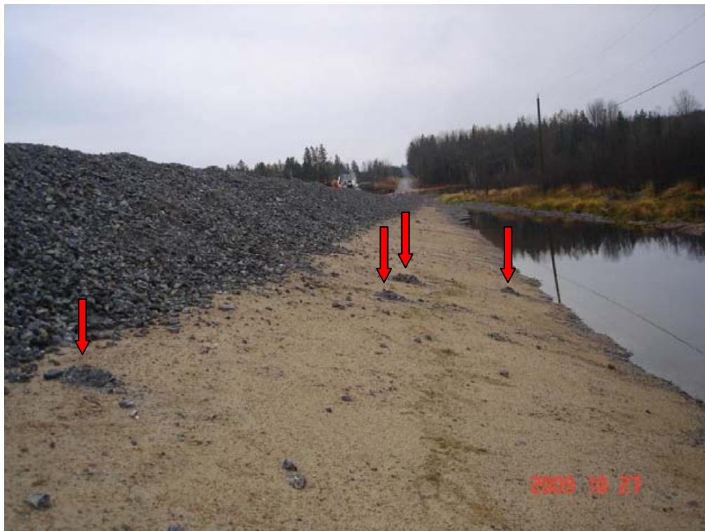
Figure E8 – More sand boils on north SSM slope (looking west)
