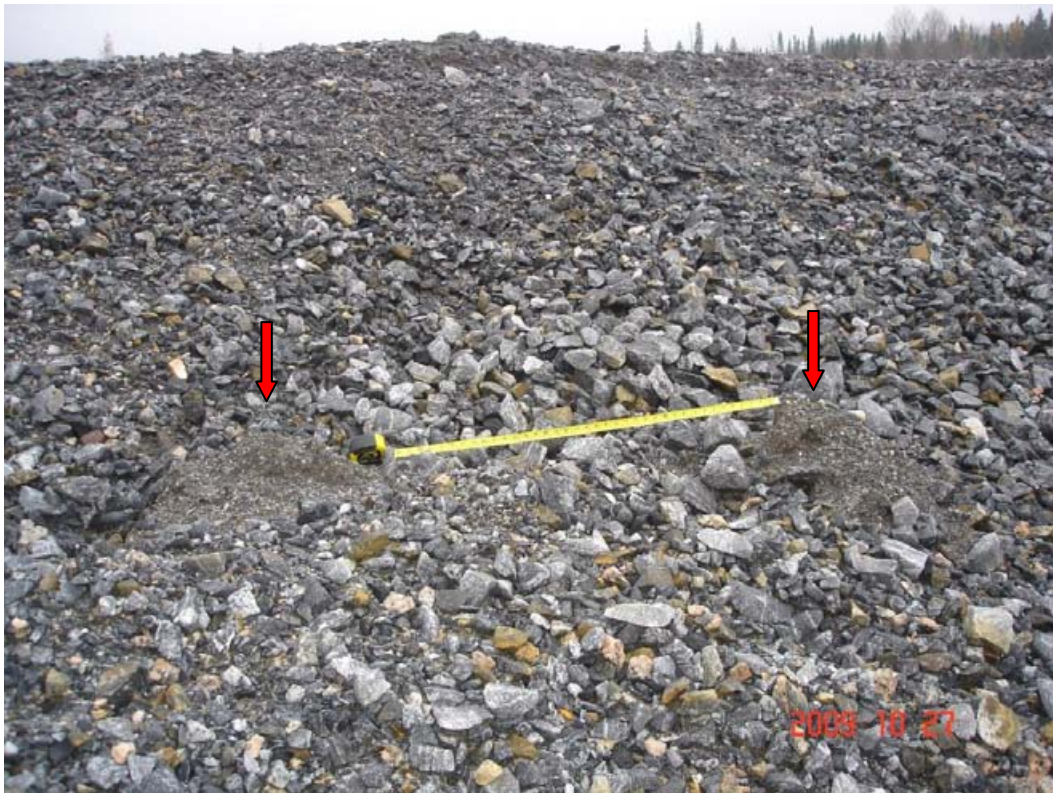
Figure E10 – More sand boils on south Granular B Type 2 Surcharge slope
