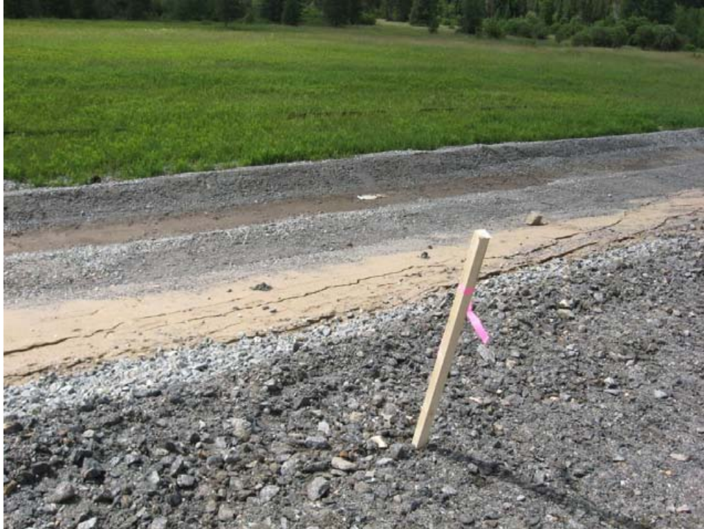
Figure E5 –South toe bulge (looking south west)
