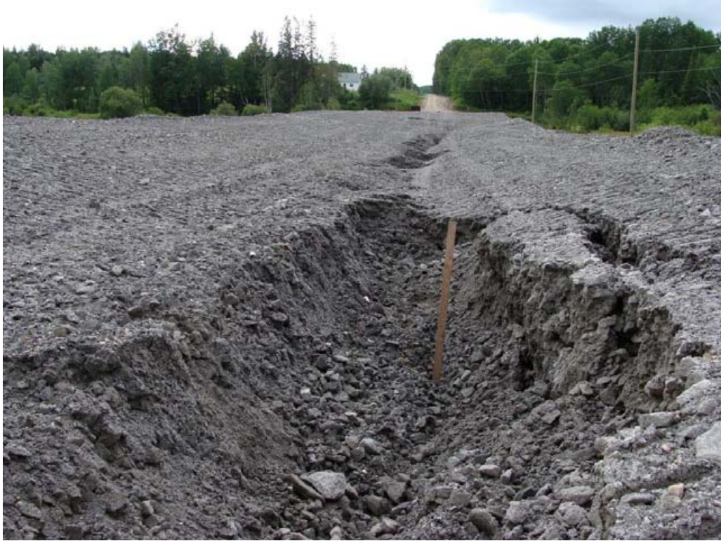
Figure E3 – Tension Cracks at the top of embankment (looking west)
