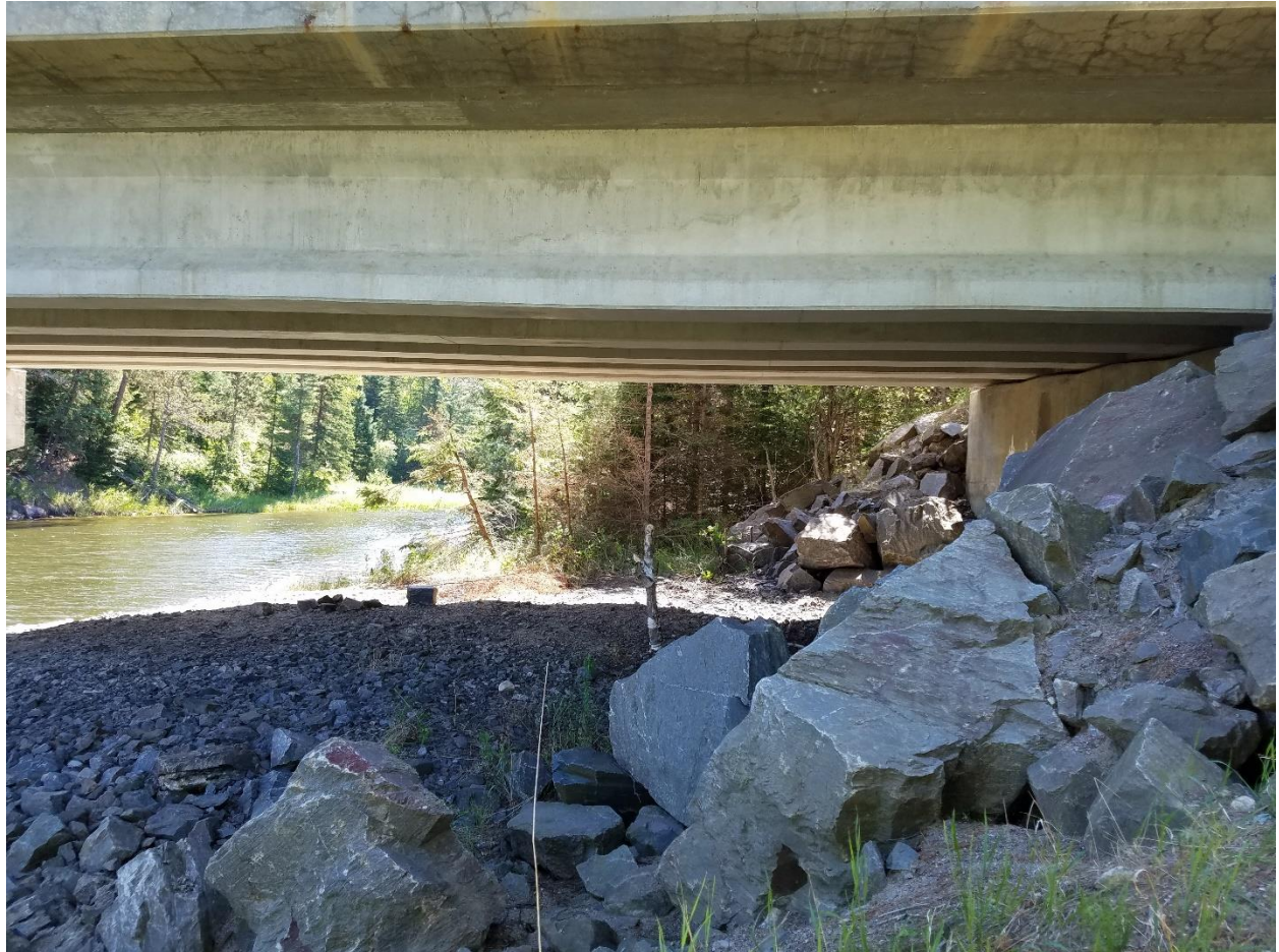
Photograph # 4 – Rock Fill at West Abutment (July 2018)
