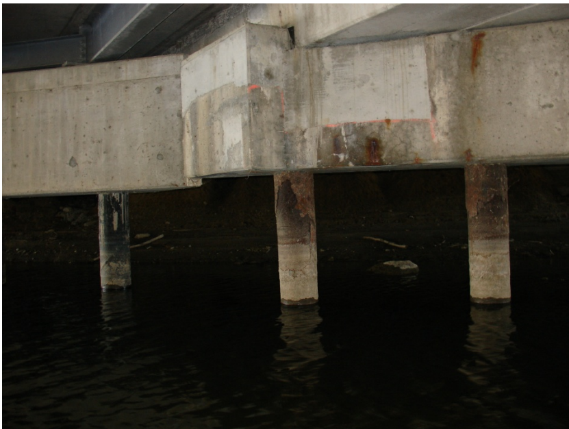
Bridge 1 - Typical deterioration of east piles
