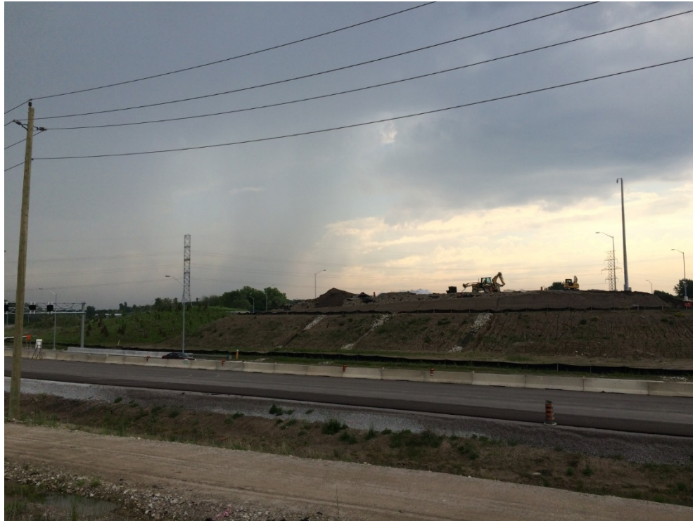
Photograph 1: Bridge Site B-1 - Construction of east approach embankment.
