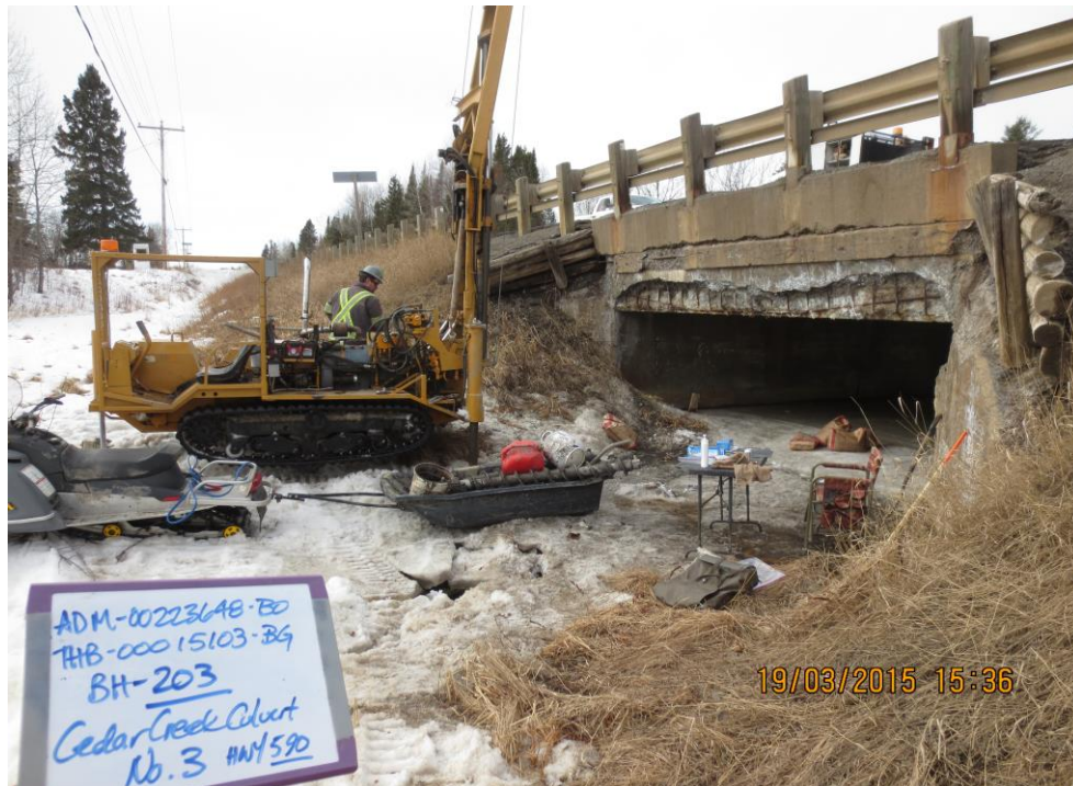
Photo 2. Outlet of existing culvert at south side of Highway 590, deterioration observed
