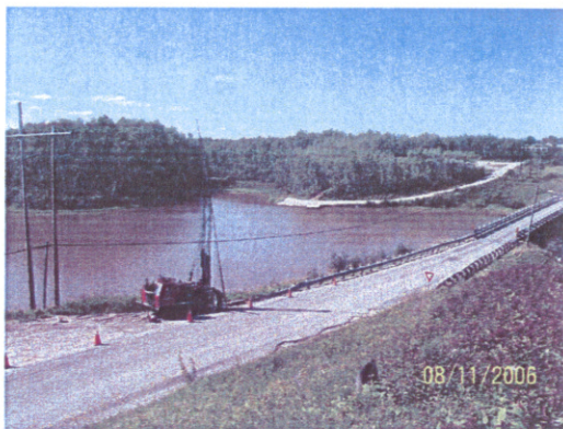
Photographs 5 & 6 - Deployment of the drilling rig on the south side of the bridge with traffic control & safety measures in place along the highway
