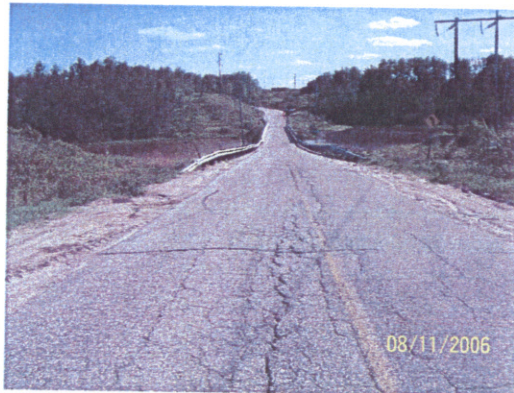
Photographs 9 & 10 - Existing pavement condition along the approach embankment
