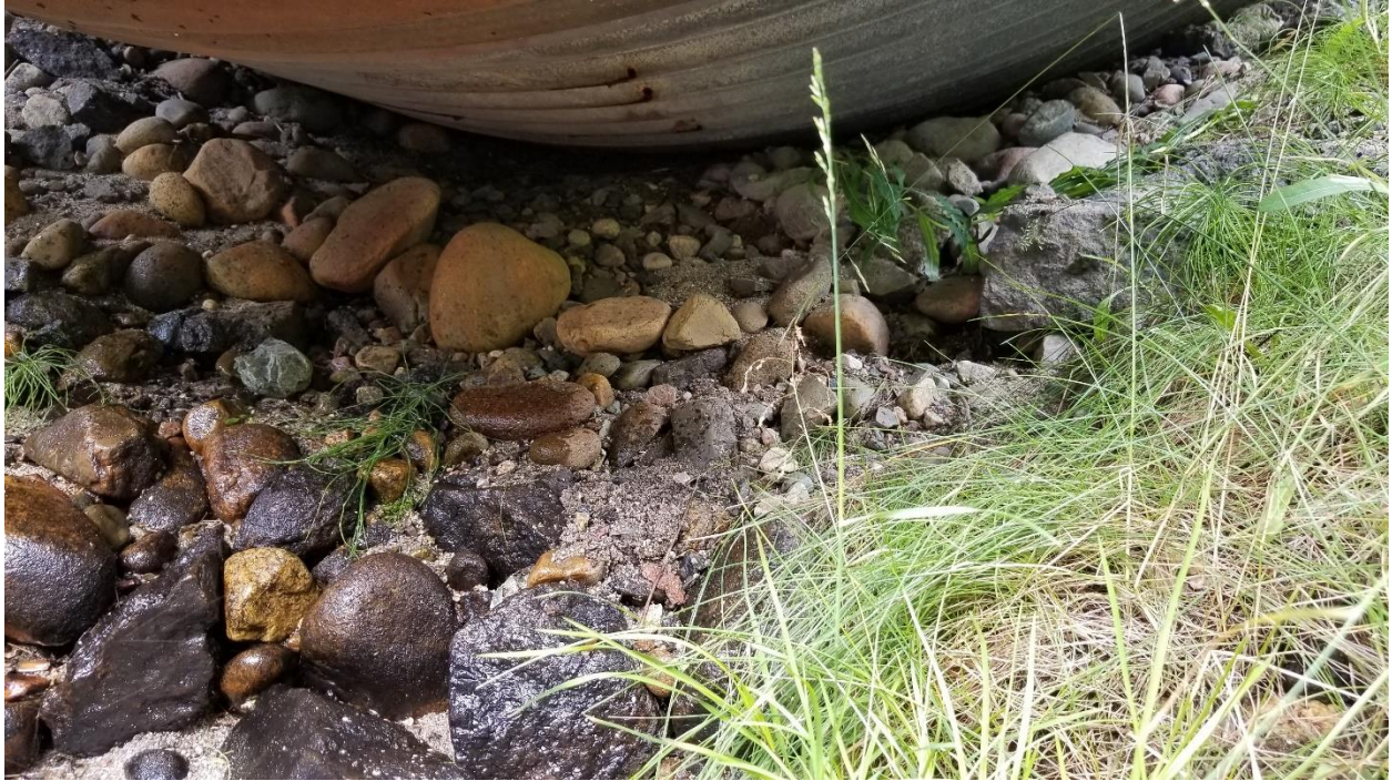
Photo 8: Outlet of culvert resting on sand, gravel and cobbles (possibly fill) (Date taken: August 23, 2017)
