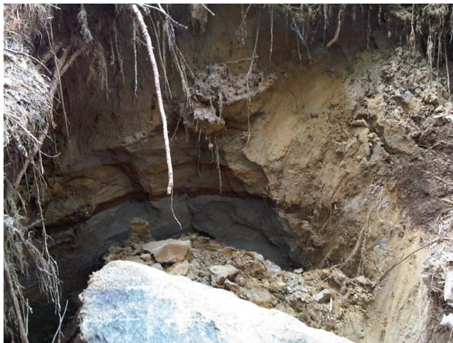
Photo 5. Sinkhole in the east embankment
