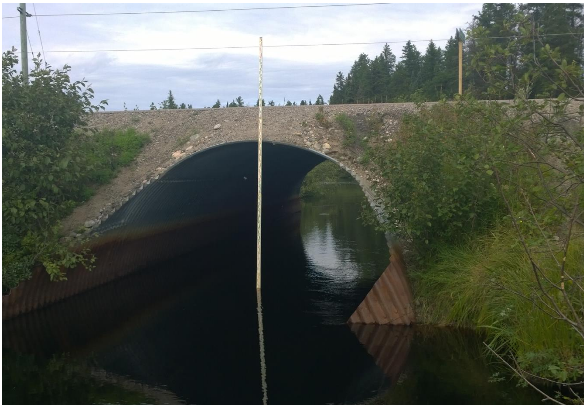
Photo 5. Inlet of Donnegana River Culvert, South Side of Hwy 560.
