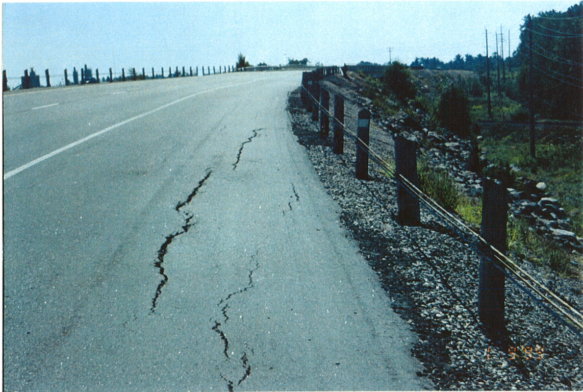
DISTRESS CRACKS IN THE VICINITY OF CHAINAGE 15 + 000 ( VIEW LOOKING SOUTH )
