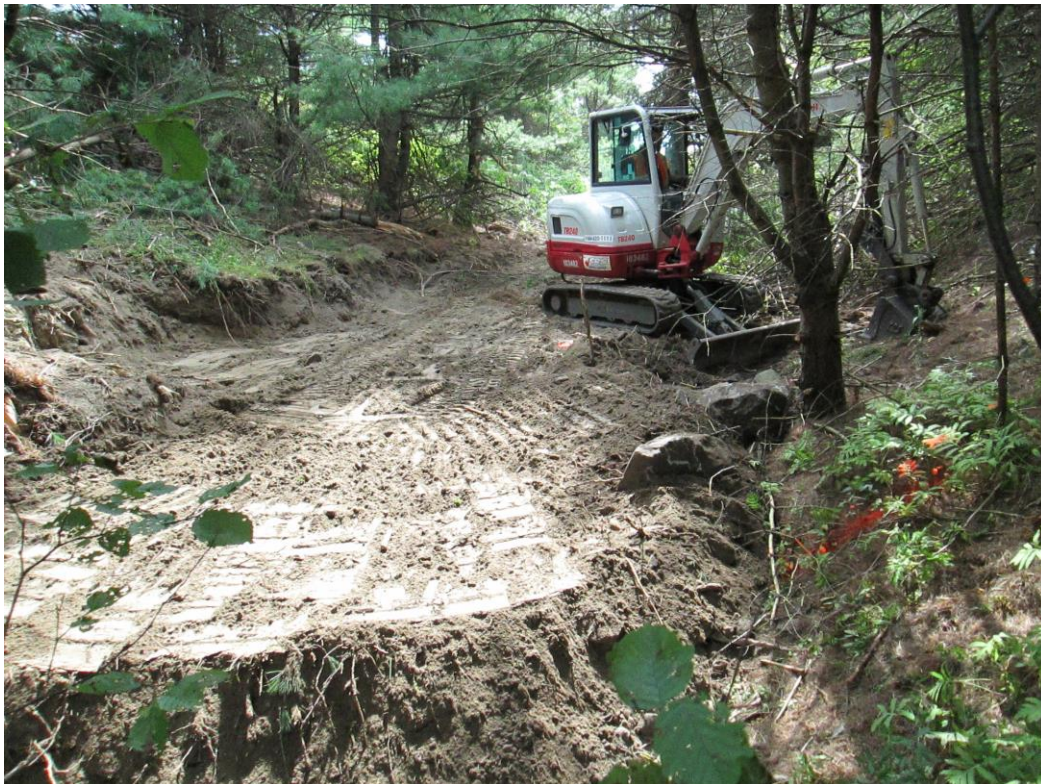
Photo 8: Building platform for HDD and access for drill rig for BH-5
