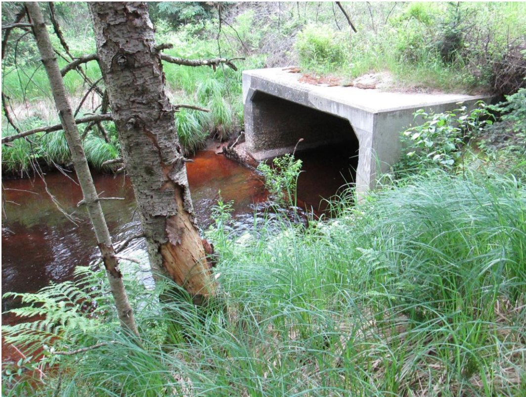
Photo 11: Existing Box Culvert outlet
