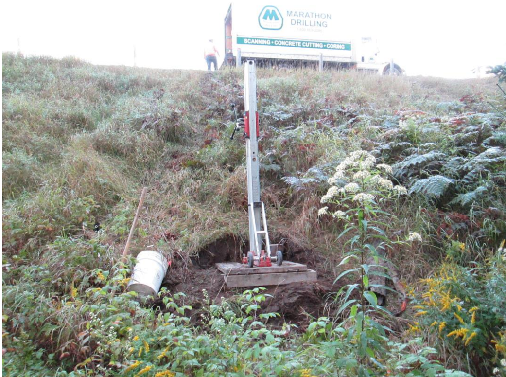
Photo 15: Portable drill at BH-7 location looking east from existing culvert outlet
