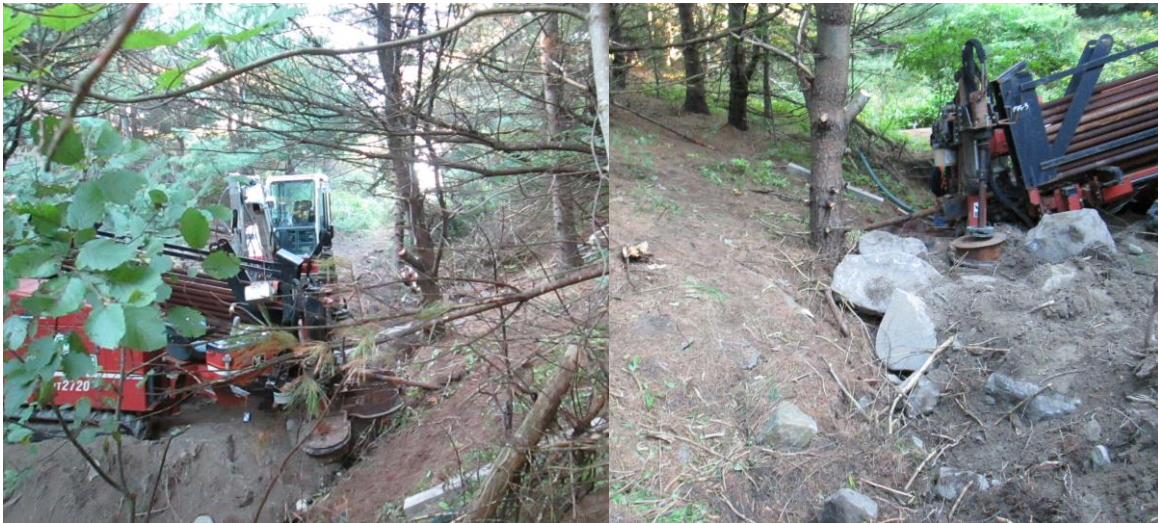
Photo 13: Starting point of horizontal probe hole at inlet side
