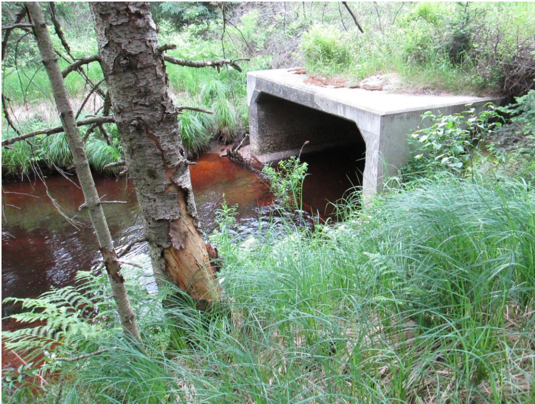
Photo 11: Existing Box Culvert outlet
