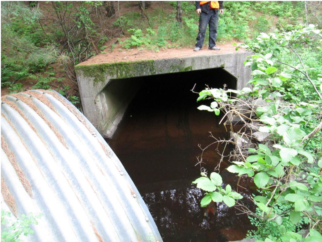
Photo 10: Existing Box Culvert inlet and outlet of CSP culvert
