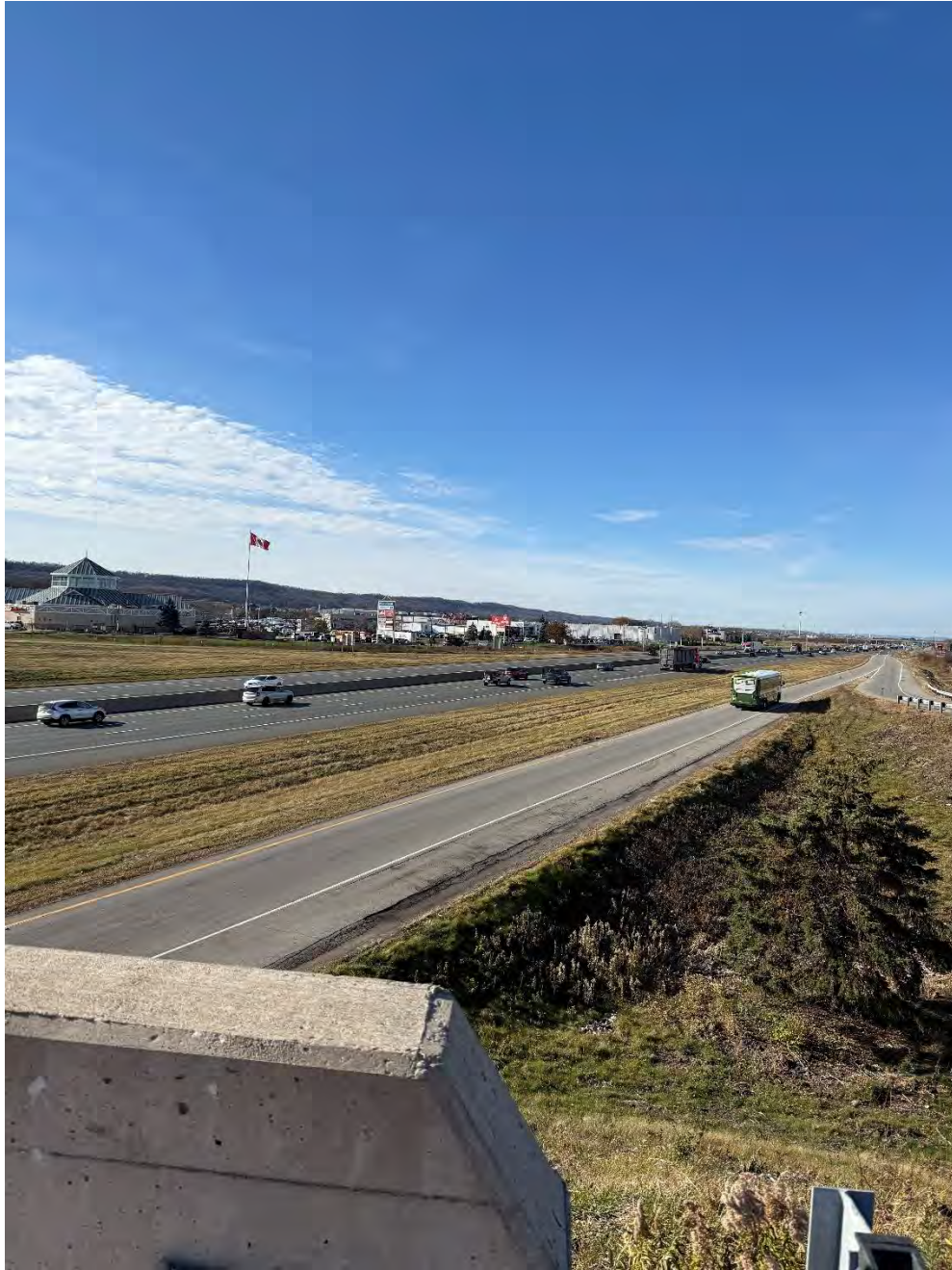
Photograph 2: Casablanca Boulevard Bridge overlooking QEW, looking West
