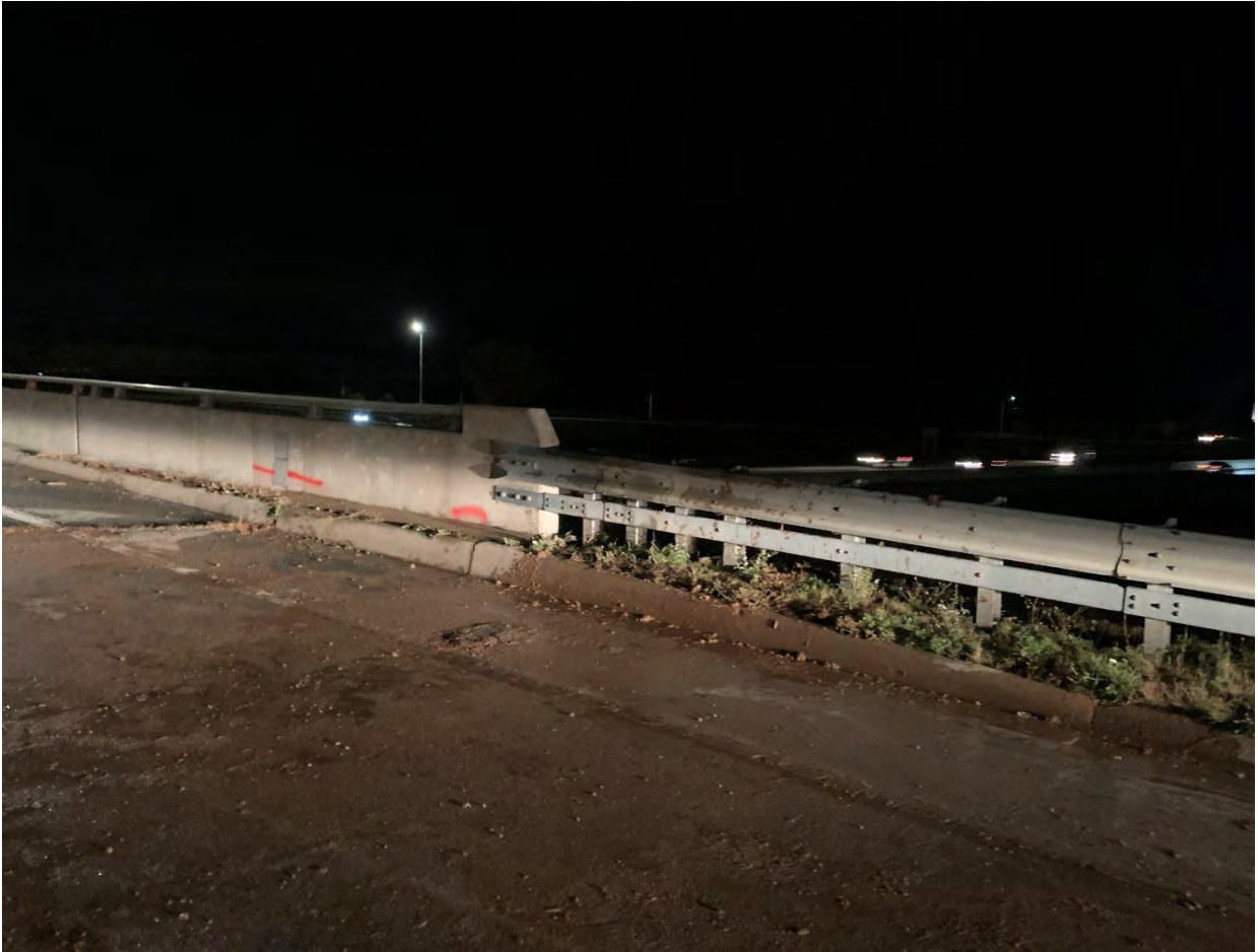
Photograph 4: Borehole 25-01 after competition, looking East
