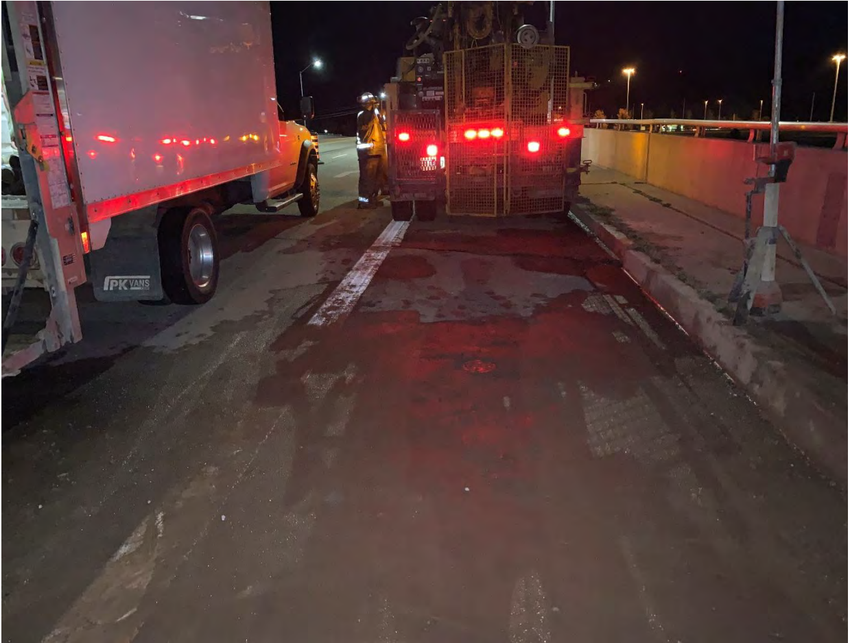
Photograph 5: Borehole 25-02 after completion, looking west
