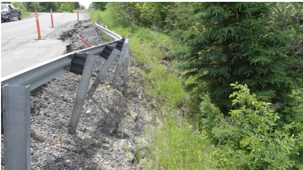
Photograph 2. 2022 Slope instability on Highway 658, facing south, July 7, 2022
