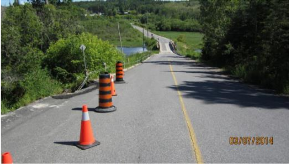
Photo 9 (Looking North): July 3, 2014 – Leaning Power Poles 2014 Slope Instability
