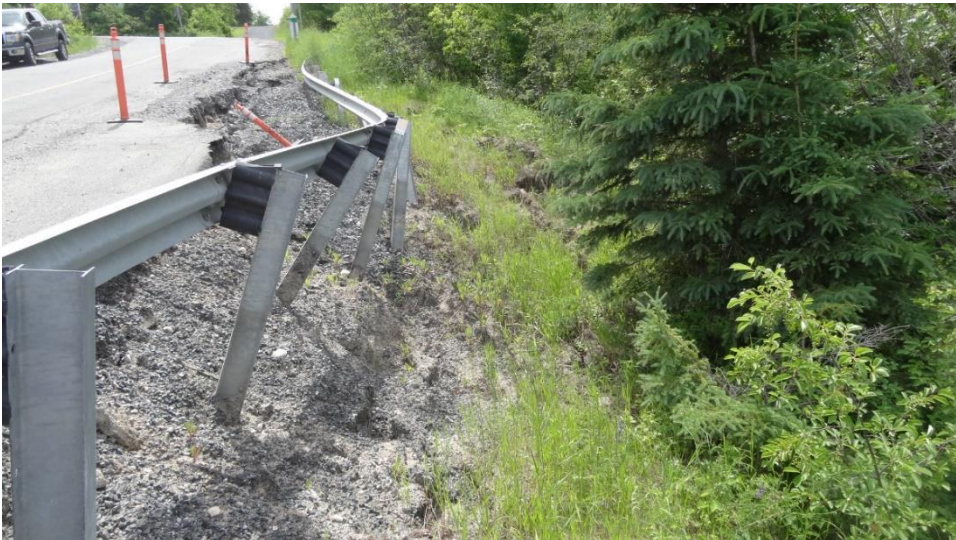
Photo 6 (Looking South): July 7, 2022 – Highway 658 West Embankment Slope Instability
