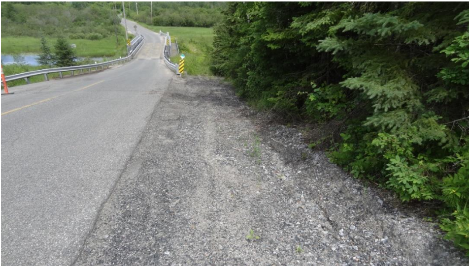
Photo 11 (Looking North): July 7, 2022 – Highway 658 East Shoulder Surficial Drainage Erosion
