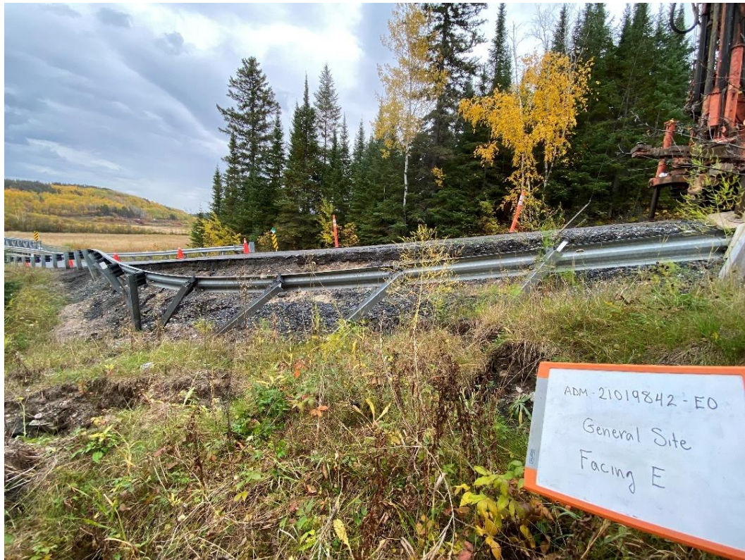
Photograph 5. 2022 Slope instability on Highway 658, facing east, October 2022
