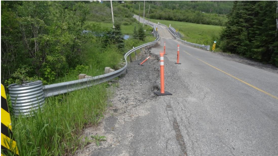
Photograph 1. 2022 Slope instability on Highway 658, facing north, July 7, 2022
