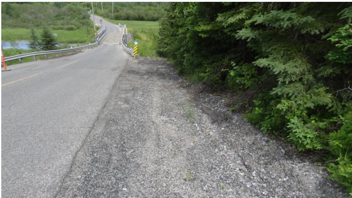
Photograph 4. Highway 658 east shoulder surficial drainage erosion, facing north, July 7, 2022
