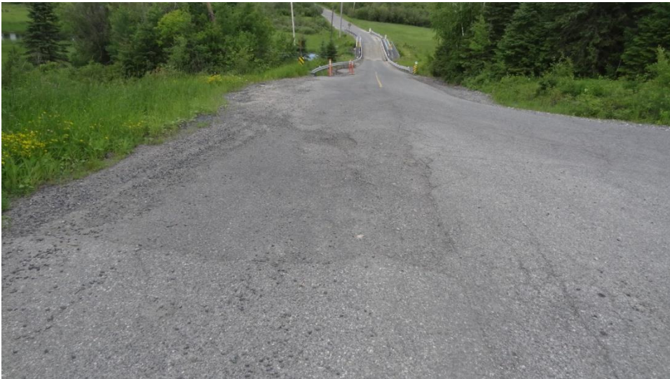
Photo 17 (Looking North): July 7, 2022 – Asphalt Repair Patch Adjacent to 2014 Instability Area
