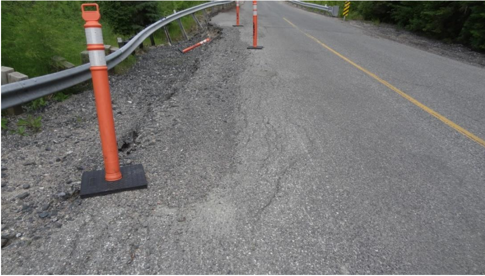
Photo 10 (Looking North): July 7, 2022 – Highway 658 West Shoulder Gravel-Treated Roadway Repair
