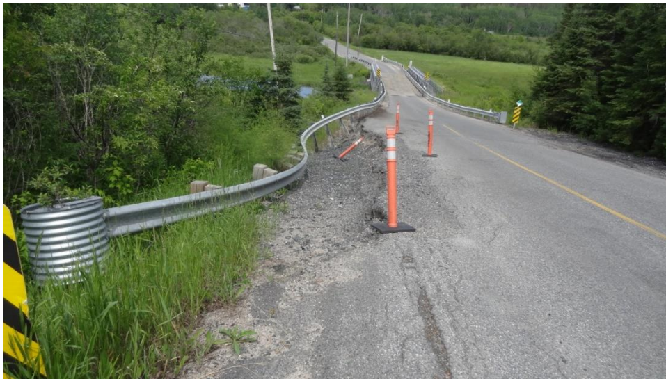
Photo 1 (Looking North): July 7, 2022 – Highway 658 Slope Instability
