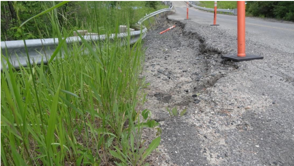
Photo 3 (Looking North): July 7, 2022 – Slope Instability Head Scarp Parallel to Highway 658
