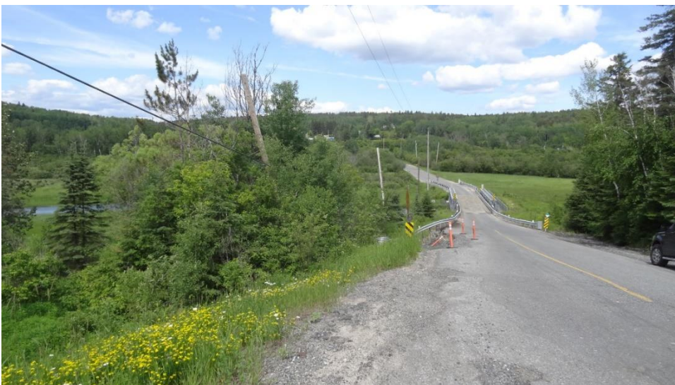
Photo 8 (Looking North): July 7, 2022 – Leaning Power Poles 2022 Slope Instability
