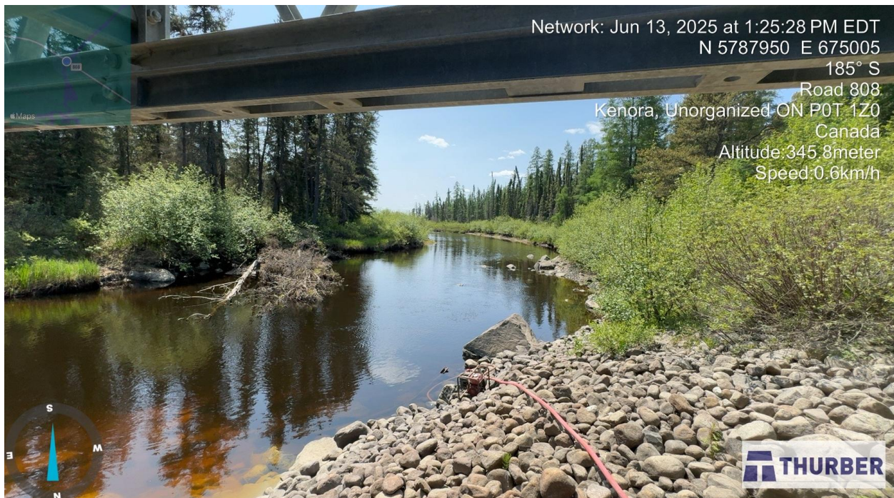
Photo 16: Looking south at the river, below the bridge (June 13, 2025).
