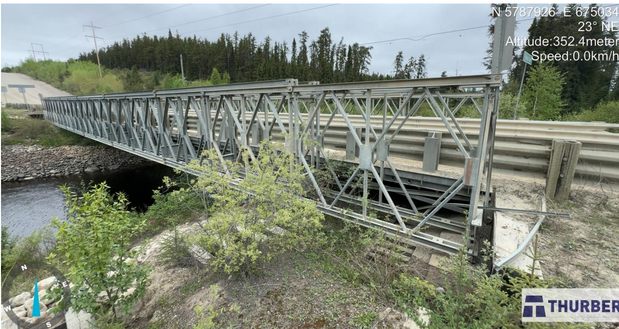
Photo 6: Looking north at Pineimuta River modular bridge (June 11, 2025).
