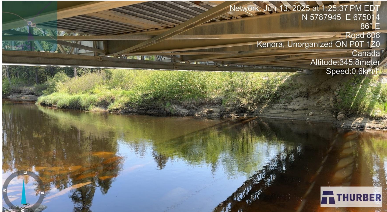
Photo 17: Looking at the river, below the bridge (June 13, 2025).
