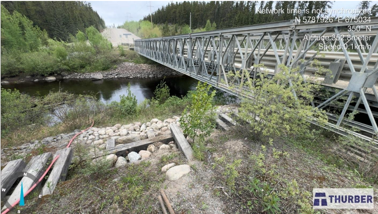
Photo 5: Looking north at Pineimuta River and modular bridge (June 11, 2025).
