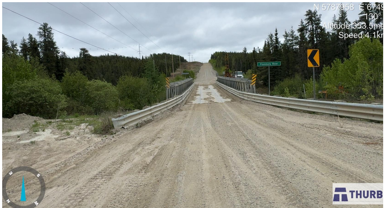
Photo 2: Looking southeast at existing east structure (June 11, 2025).
