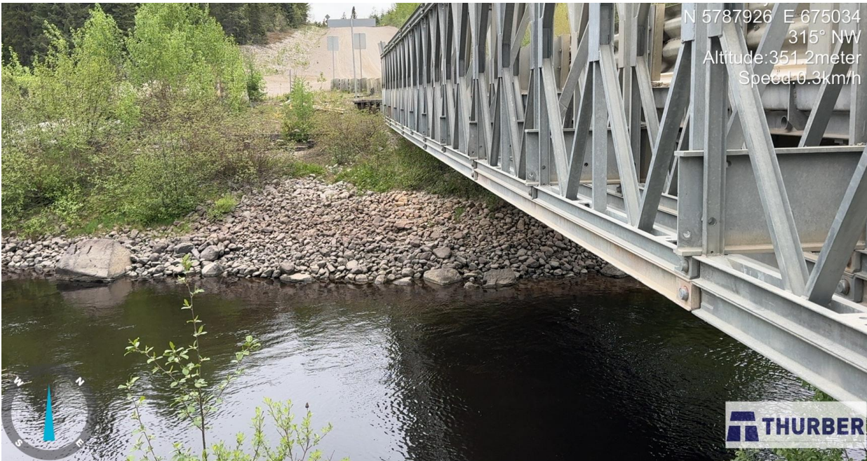
Photo 9: Looking northwest at the bridge embankment fill (June 11, 2025).
