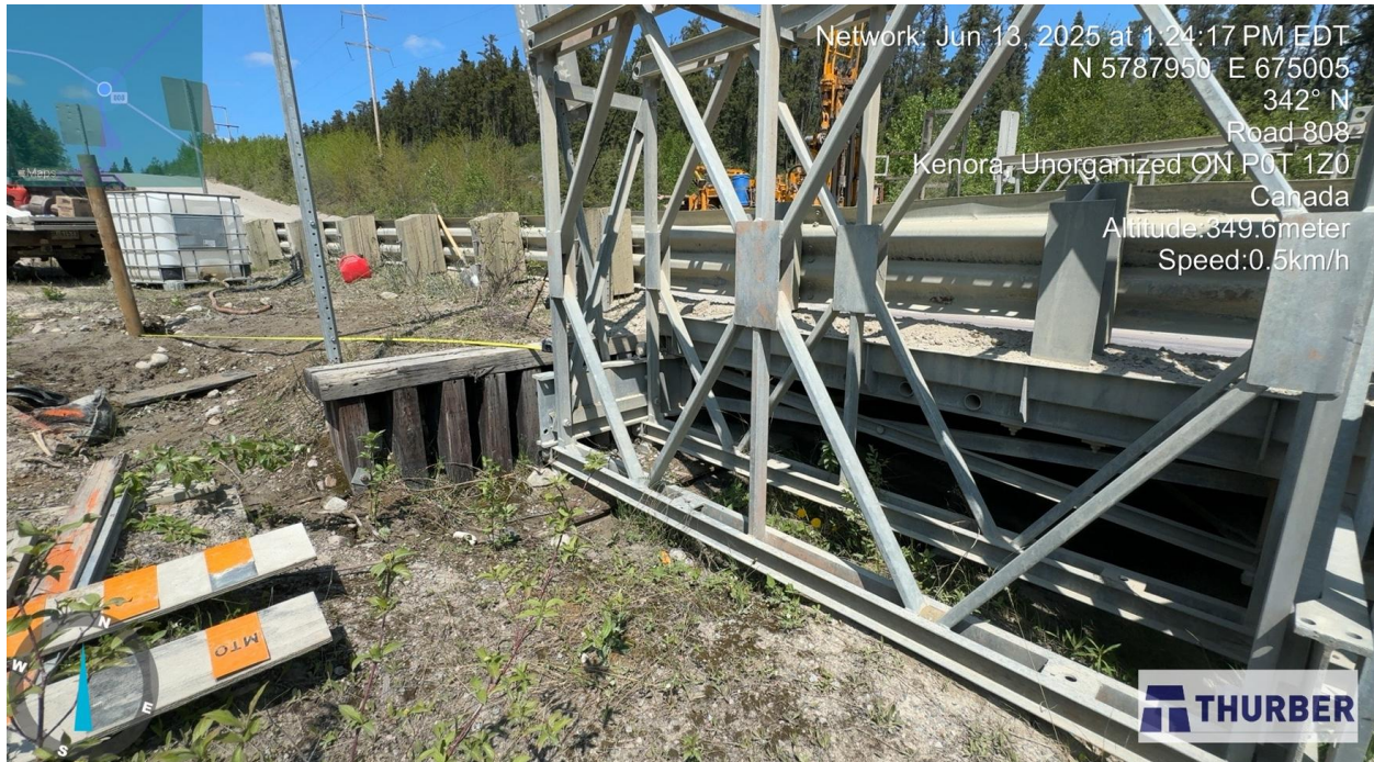
Photo 15: Looking north at the bridge approach (June 13, 2025).
