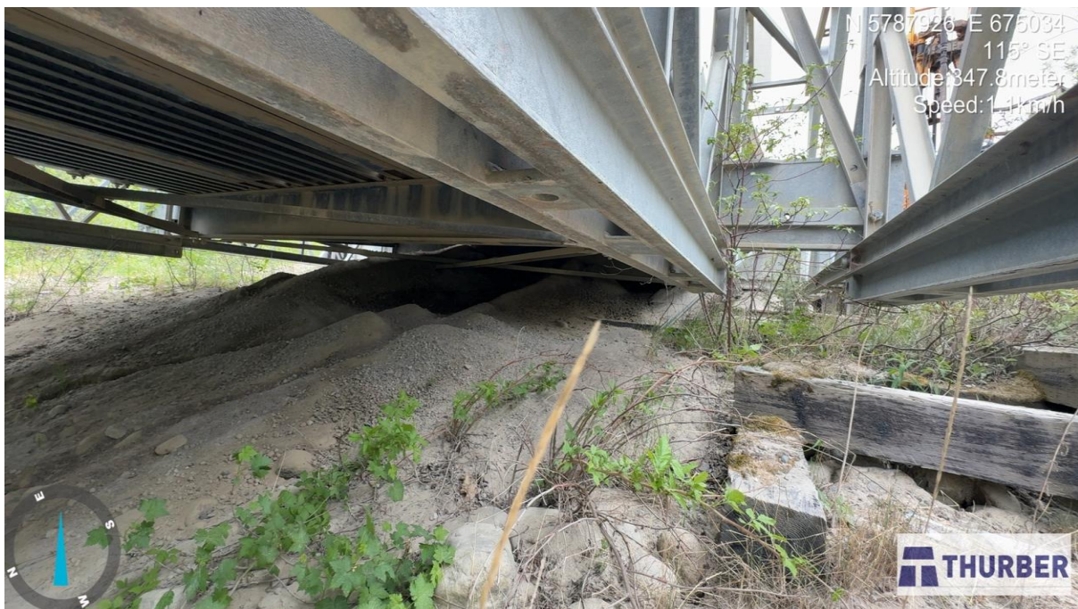
Photo 8: Looking east below the bridge (June 11, 2025).
