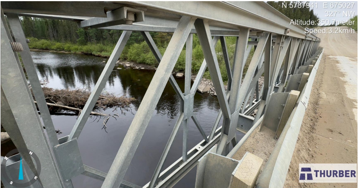
Photo 4: Looking west at Pineimuta River from modular bridge (June 11, 2025).
