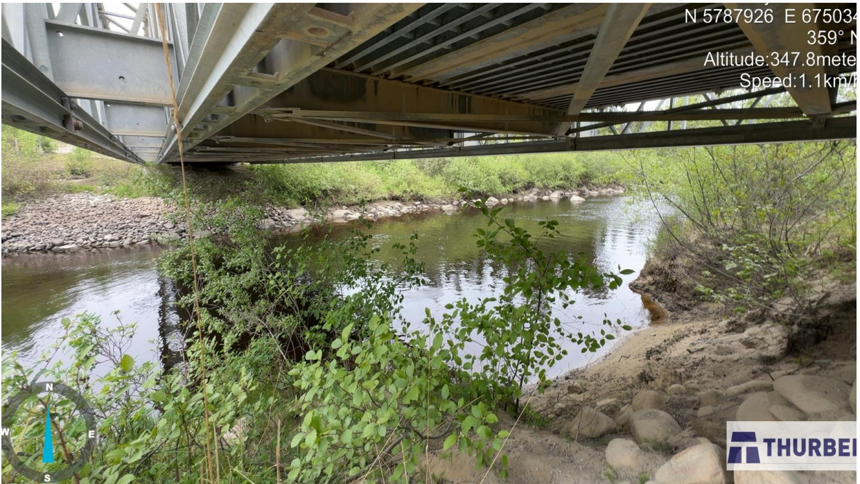
Photo 7: Looking north at Pineimuta River from under the bridge (June 11, 2025).
