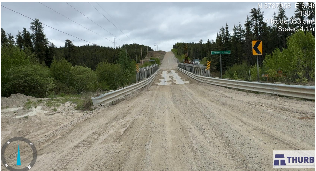
Photo 2: Looking southeast at existing east structure (June 11, 2025).
