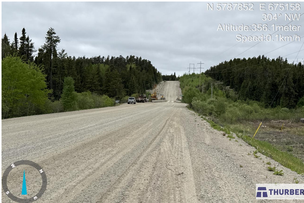
Photo 1: Looking northwest at existing bridge structure (June 11, 2025).
