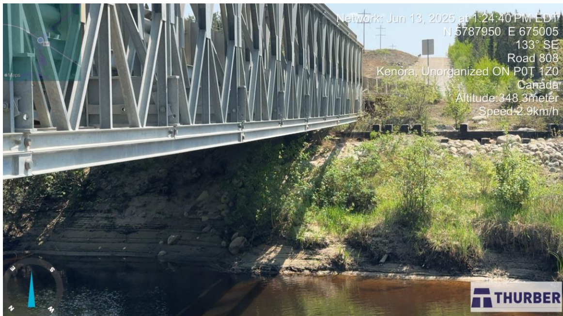
Photo 12: Looking southeast at the bridge and the embankment fill (June 13, 2025).
