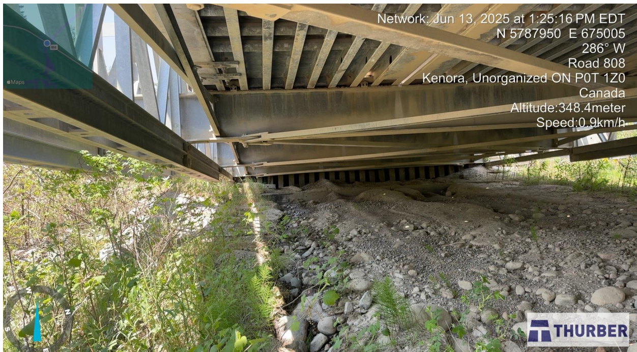
Photo 14: Looking west below the bridge (June 13, 2025).
