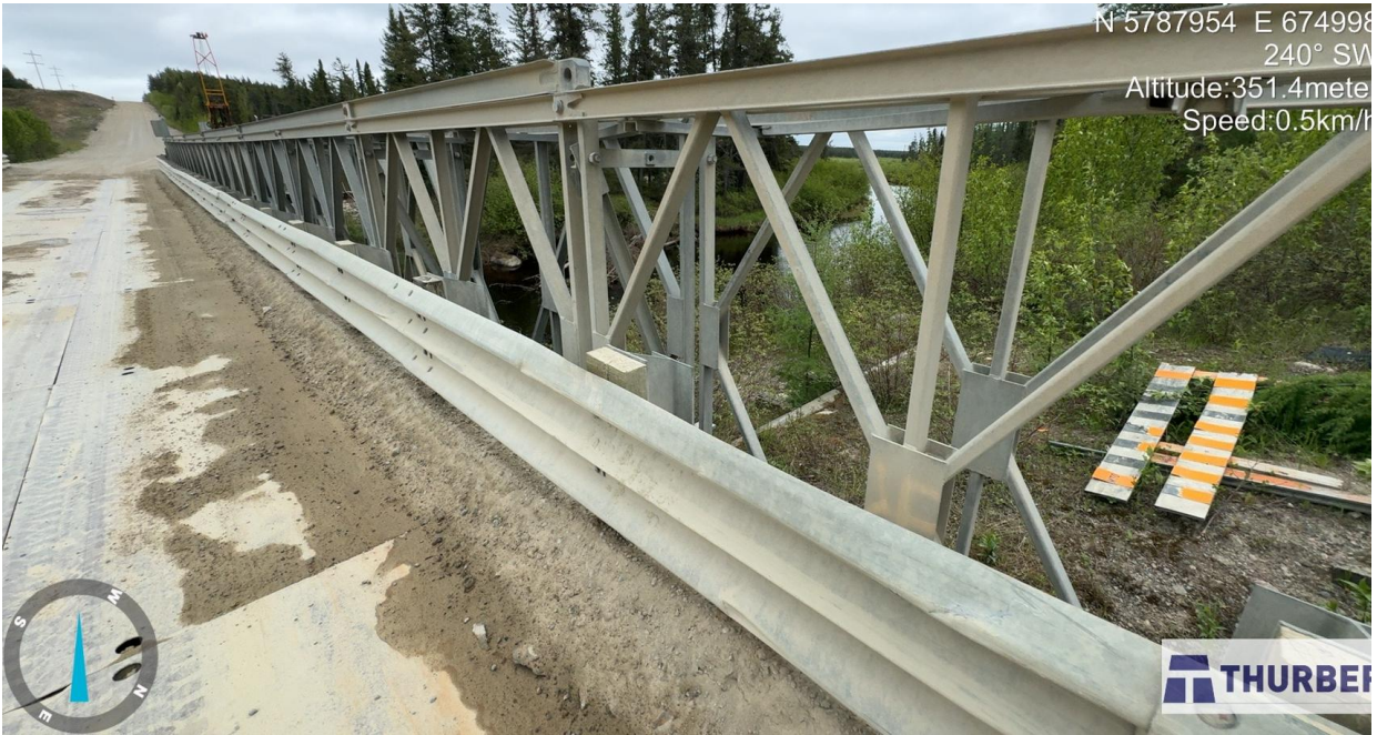
Photo 3: Looking southwest at Pineimuta River from modular bridge (June 11, 2025).
