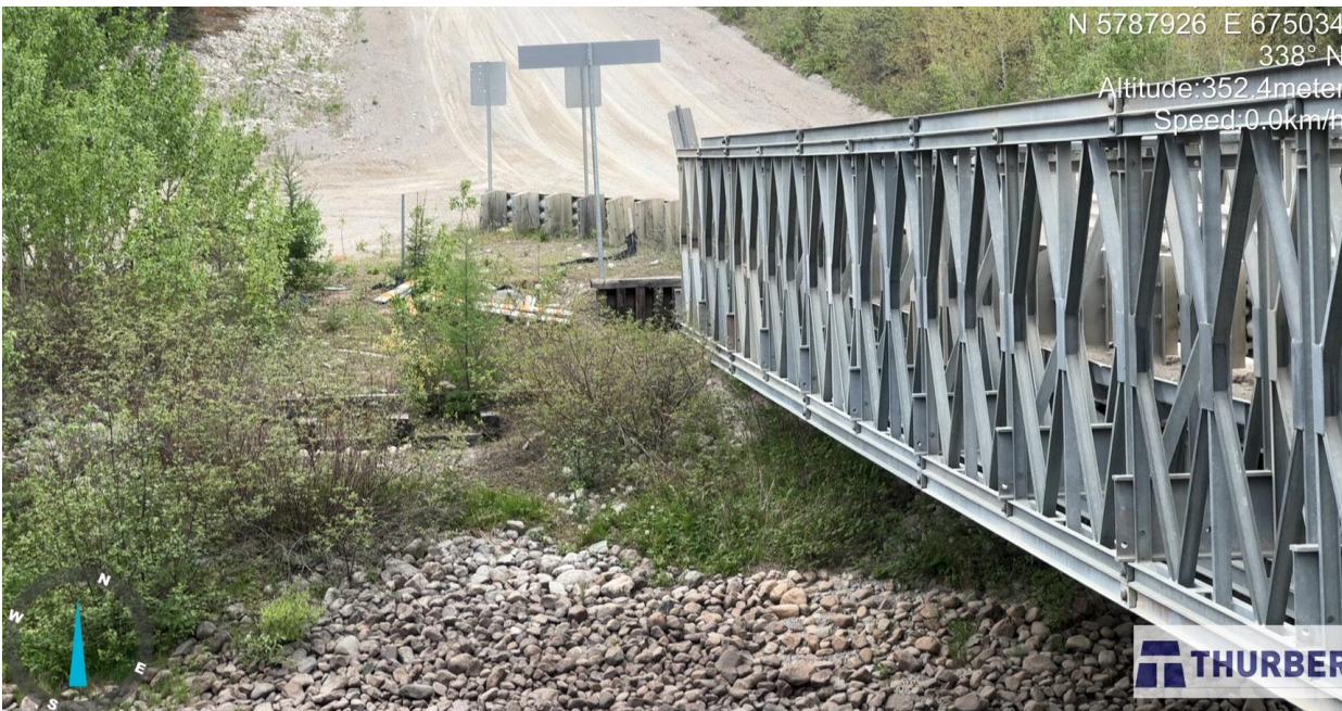
Photo 10: Looking northwest at the bridge embankment fill (June 11, 2025).
