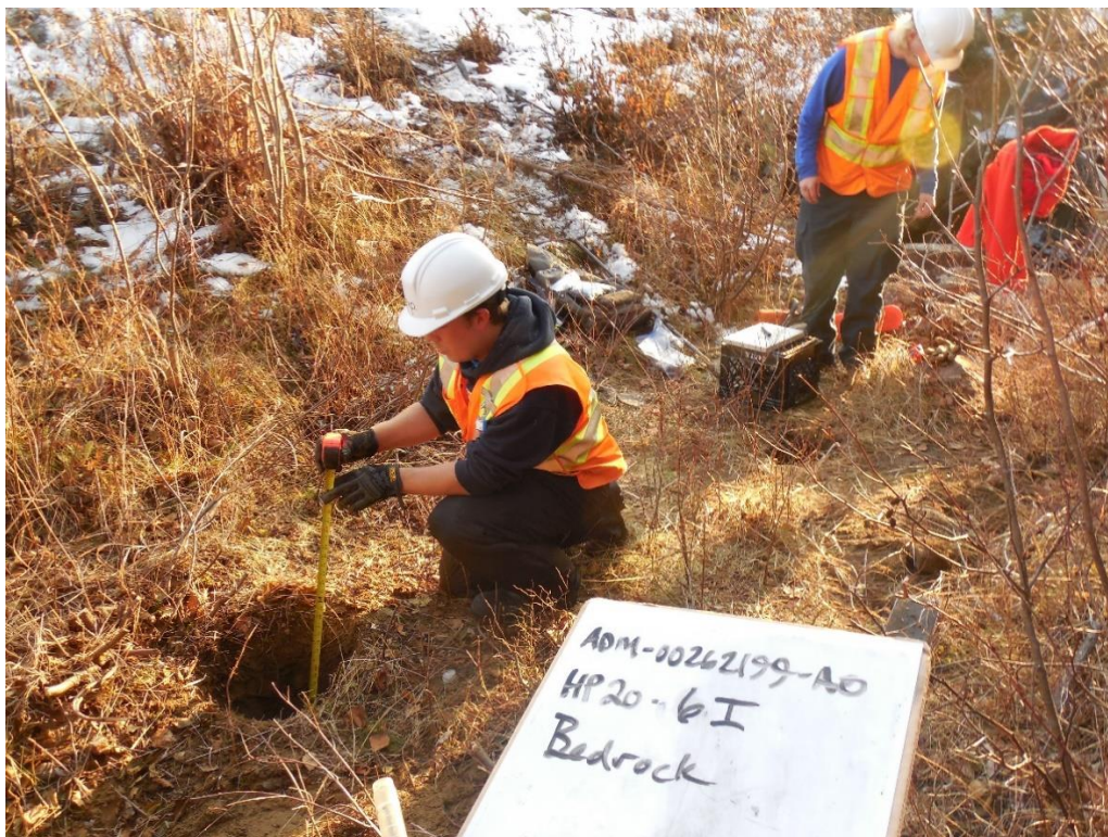
Photograph 8. Drilling hand probe hole HP20-6I, at the inlet side, November 2020
