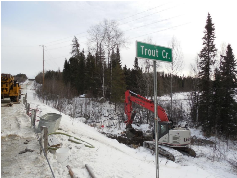
Photograph 12. View of south embankment (facing east), November 2021. Test pit TP21-1 advanced on the south side of Highway 599 and west of culverts.
