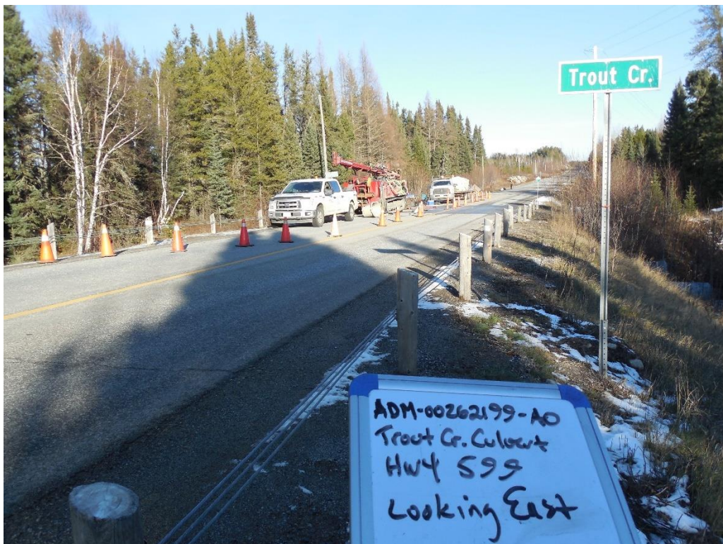
Photograph 6. Drilling borehole BH20-1 on the Highway 599 embankment (facing east), November 2020
