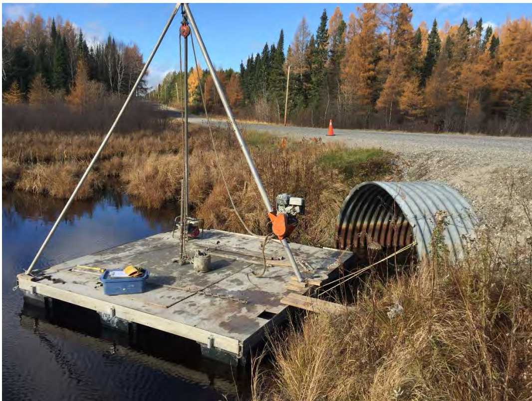
Photo 2. Raft Drilling Setup at Culvert Inlet
