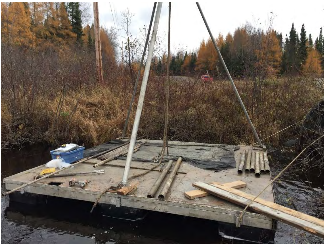
Photo 4. Raft Drilling Setup at Culvert Outlet
