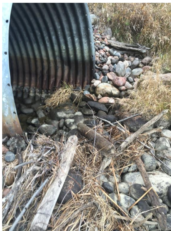
Photo 8. North CSP culvert inlet
