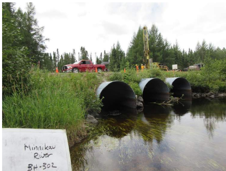
Photo 1. Existing culvert inlet on north side of highway
