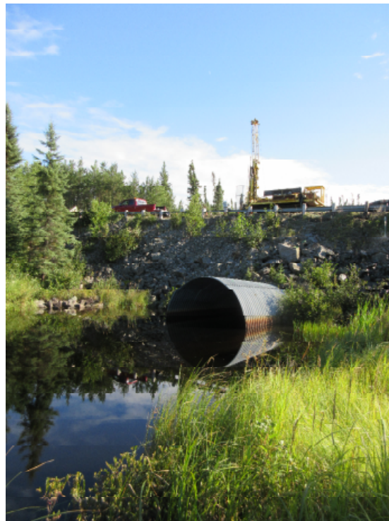
Photo 2. Existing culvert outlet on north side of highway
