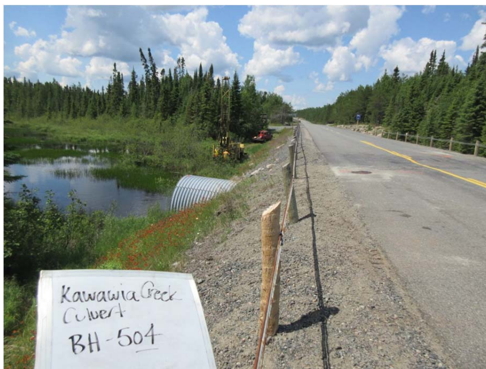
Photo 2. Existing culvert outlet on east side of highway facing south
