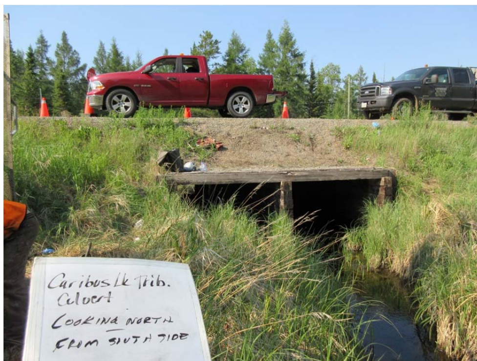
Photo 2. Existing culvert outlet on south side of highway
