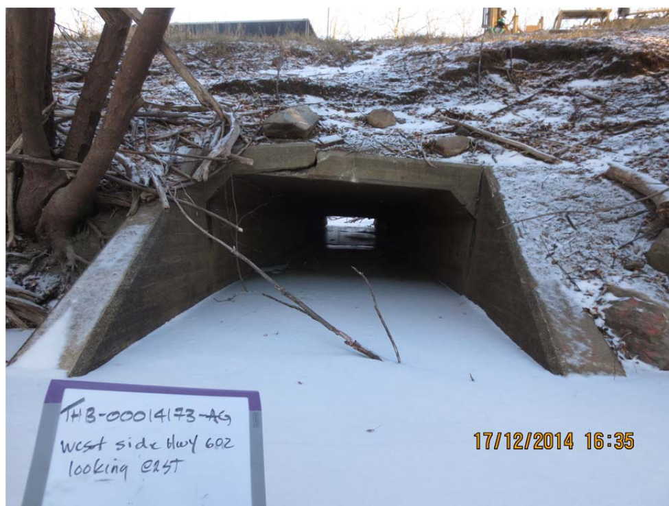
Photo 2. Outlet of existing culvert on west side of highway. Fracturing is noted.
