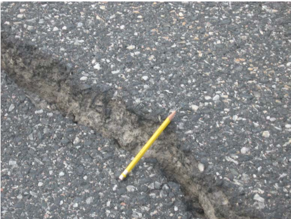
Figure 2. Relative width and depth of tension crack
