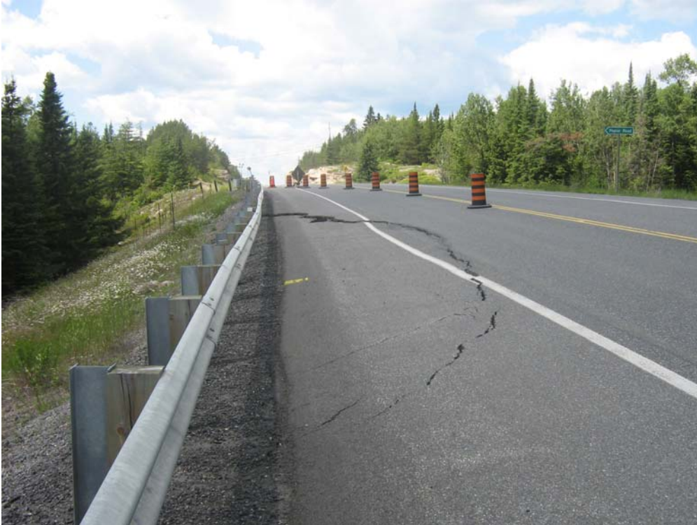
Figure 1. Tension crack along small slip
