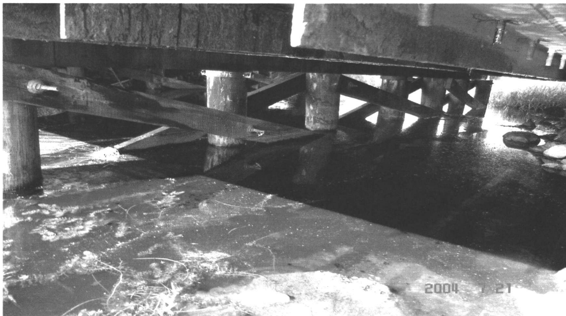
Plate 2 Existing Mather Creek # 2 timber piles.
