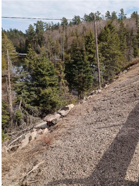
Photograph 1. Embankment slope facing southeast (April 08, 2024)
