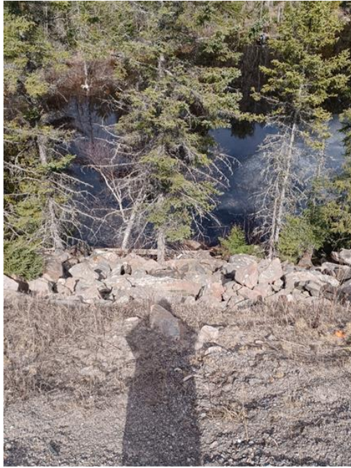
Photograph 5. East side of embankment near proposed location of BH2-1 (April 8, 2024)
