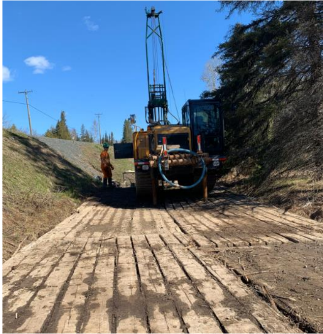
Photograph 5. East side of embankment at Borehole BH12-3 Location facing north (May 7, 2024)
