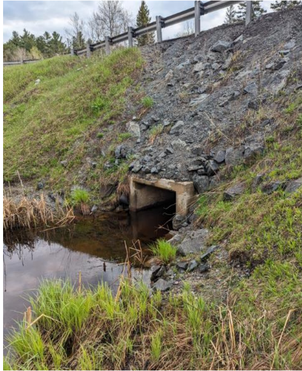
Photograph 9. Culvert outlet and west side of embankment, facing northeast (May 7, 2024)
