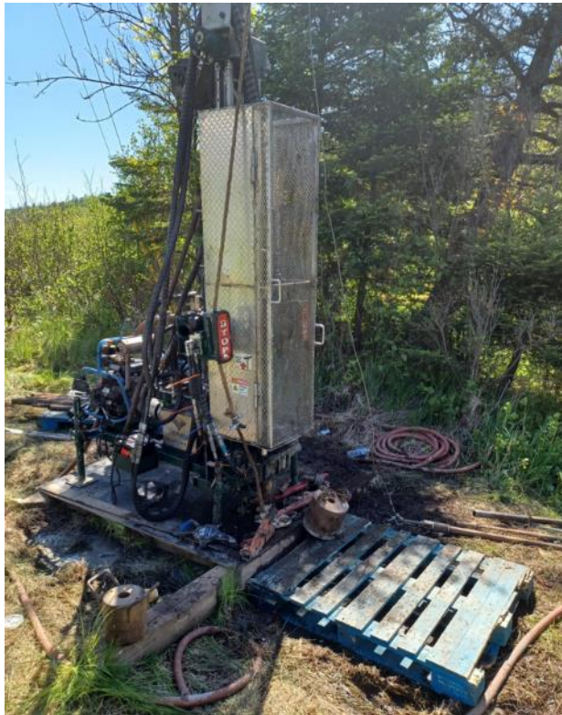
Photograph 6. West side of embankment at Borehole BH12-5 Location facing west (June 5, 2024)
