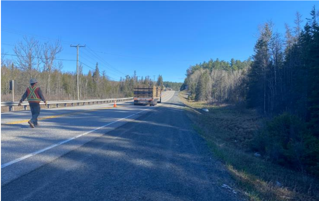
Photograph 3. Roadway surface and shoulder, embankment side slope, and ground conditions beyond embankment toe along NBL (east) side, looking north (May 6, 2024)
