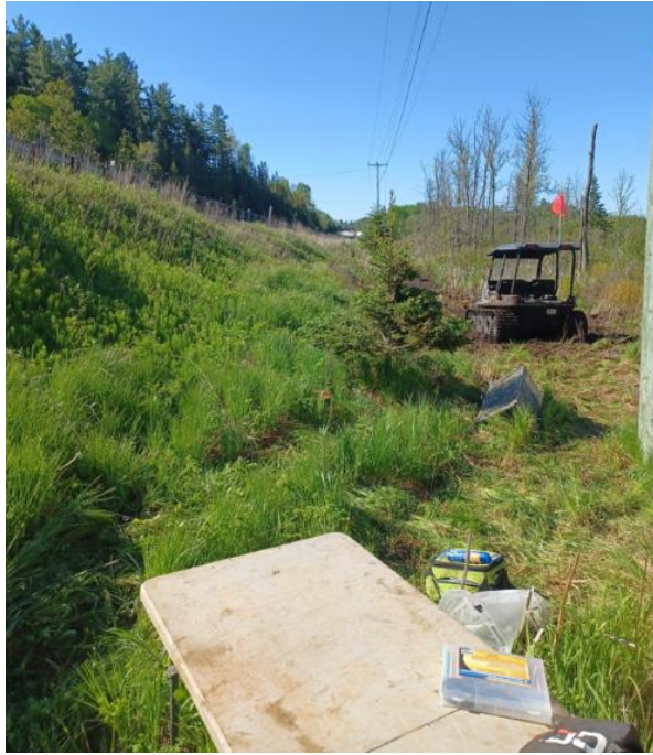
Photograph 7. West side of embankment at Borehole BH12-5 Location facing south (June 5, 2024)
