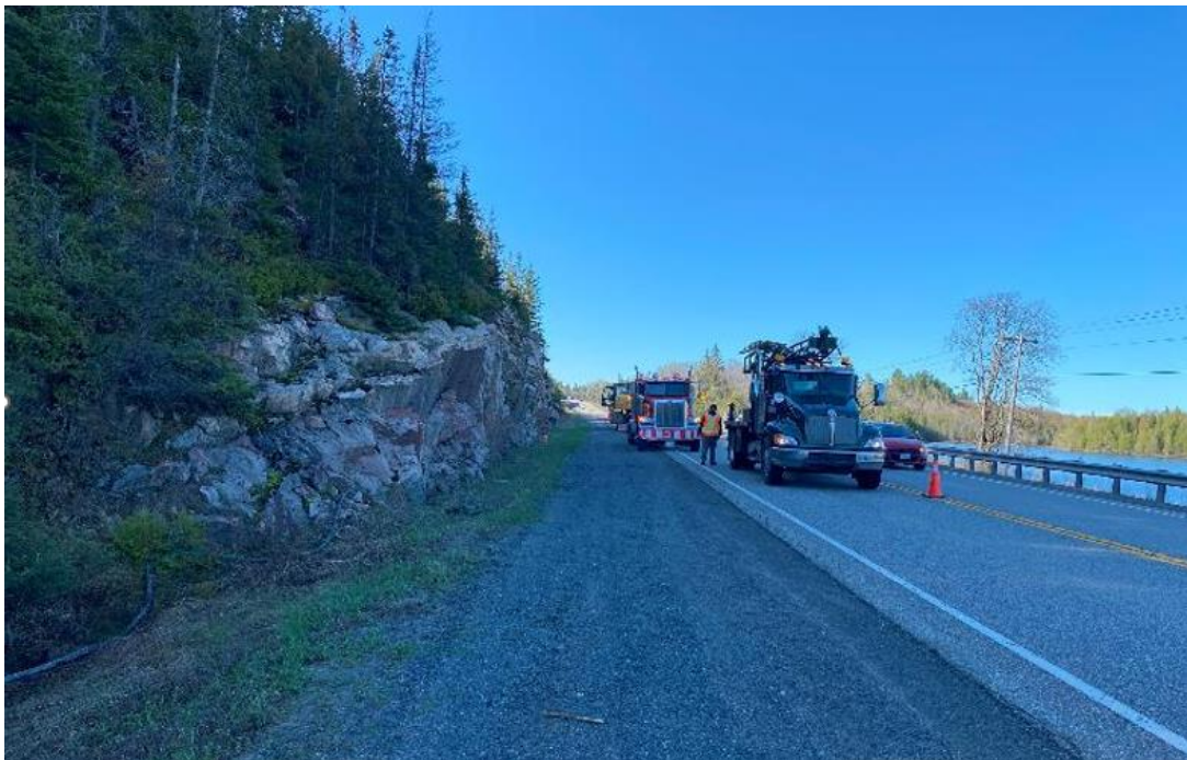
Photograph 4. Roadway surface and shoulder SBL (west) side, looking south (May 8, 2024)
