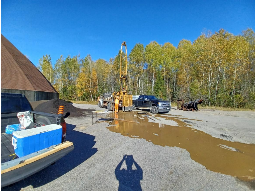
Photo 5. Shining Tree Patrol Yard – Drilling borehole 23-ST-1, facing northeast (October 3,2023)
