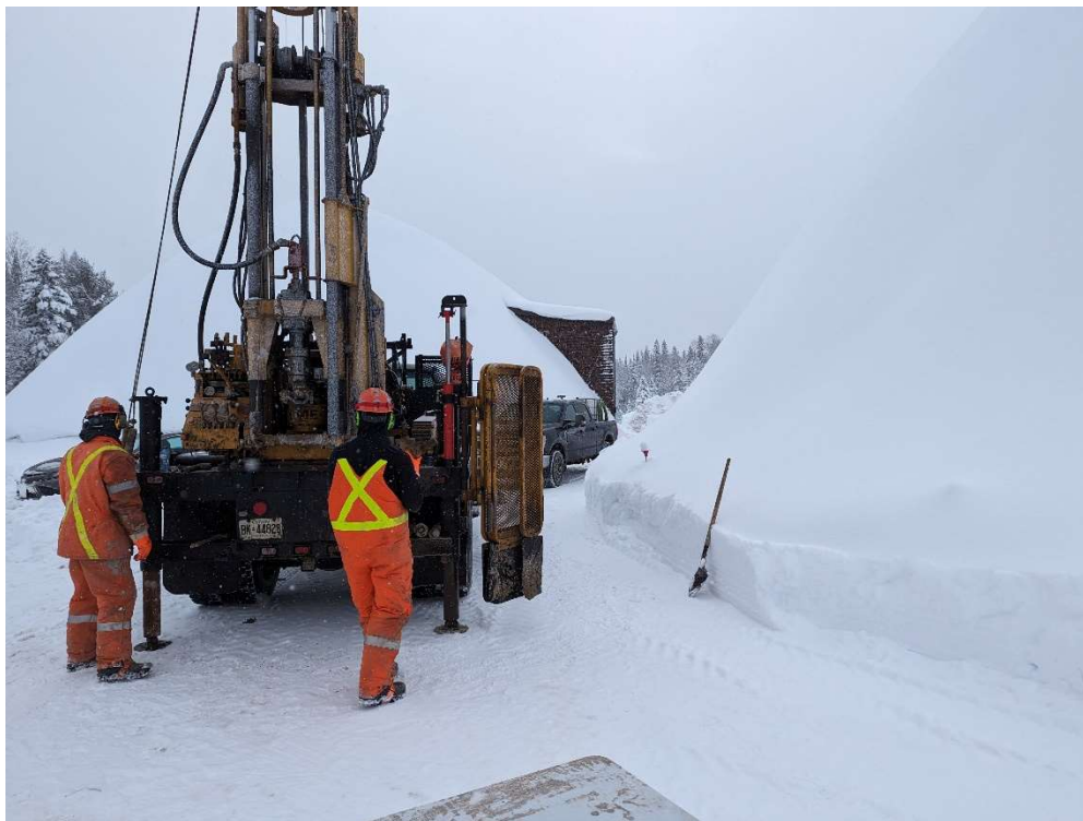
Photo 4. Dunchurch Patrol Yard – Drilling borehole BH23-D-4, facing south (January 18, 2024)
