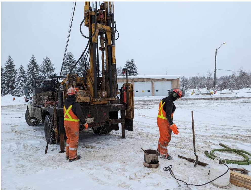
Photo 2. Dunchurch Patrol Yard – Drilling borehole BH23-D-2, facing west (January 18, 2024)
