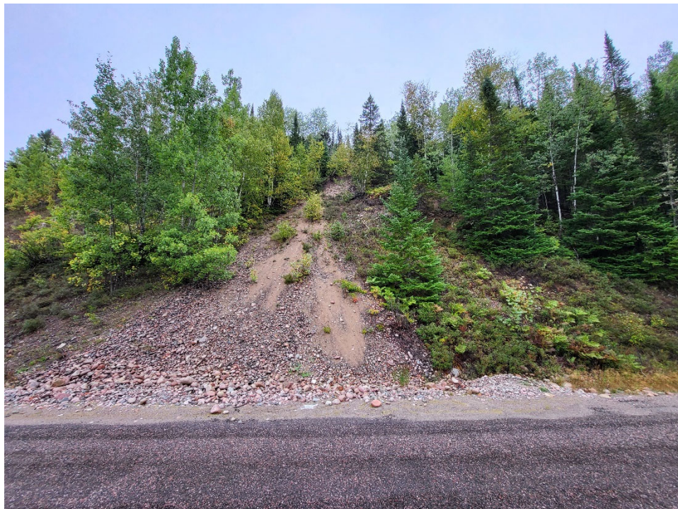
Photo 2. Active erosion near Sta. 19+350 (looking east) [taken Sept. 2022]
