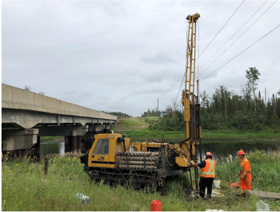
Photograph A3. West-south side of the North Driftwood River Bridge, showing drilling BH20-1
