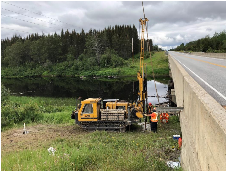
Photograph A6. East-south side of the North Driftwood River Bridge, showing drilling of BH20-5
