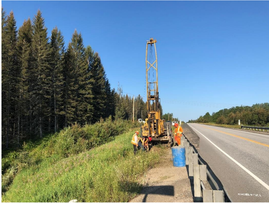
Photograph A5. West-south side of the North Driftwood River Bridge, showing drilling BH20-3
