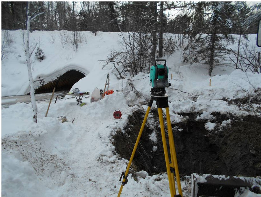
Photo 4. Site setup showing the location of the excavation and survey equipment in relation to toe of highway embankment slope and culvert/creek alignment.
