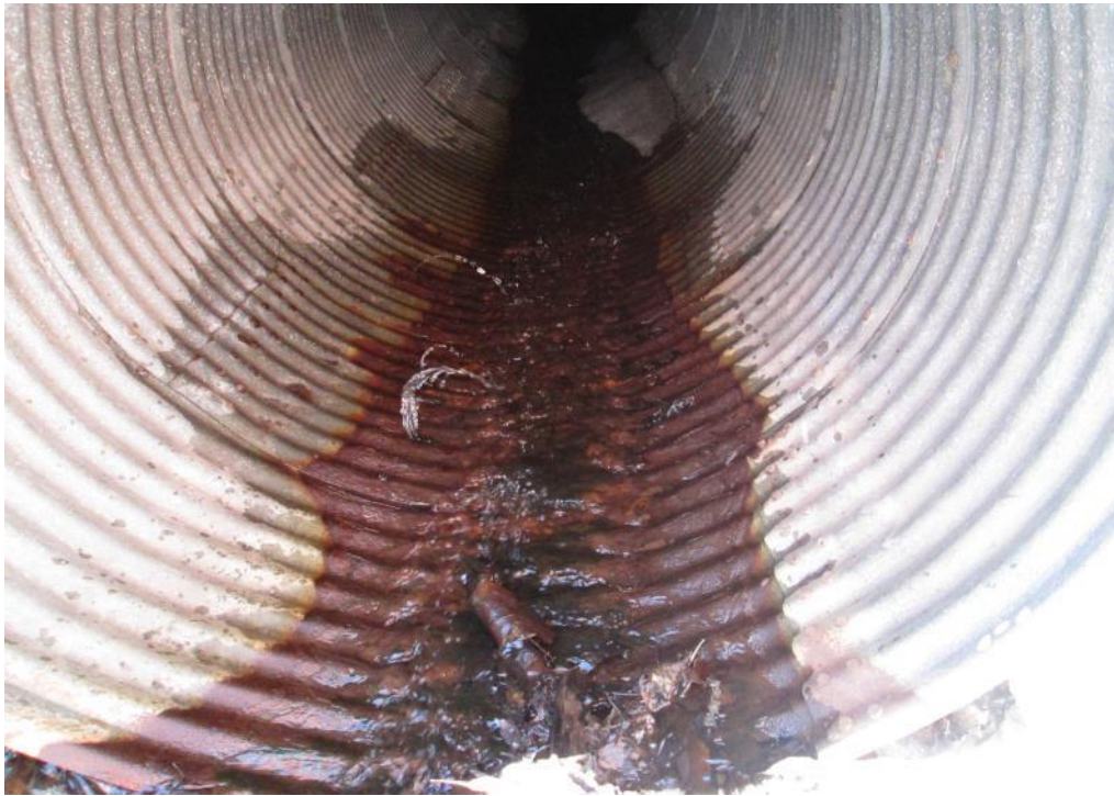
Photo 13: Deterioration of culvert at inlet
