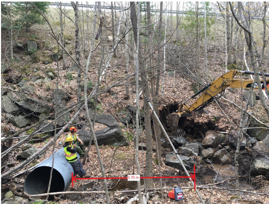
Photo 23: Test pit TP4 at the toe of the east embankment side, beginning of excavation
