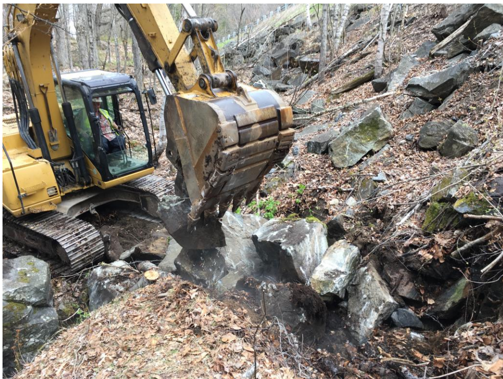
Photo 20: Test pit TP3 at the toe of west embankment slope, beginning of excavation
