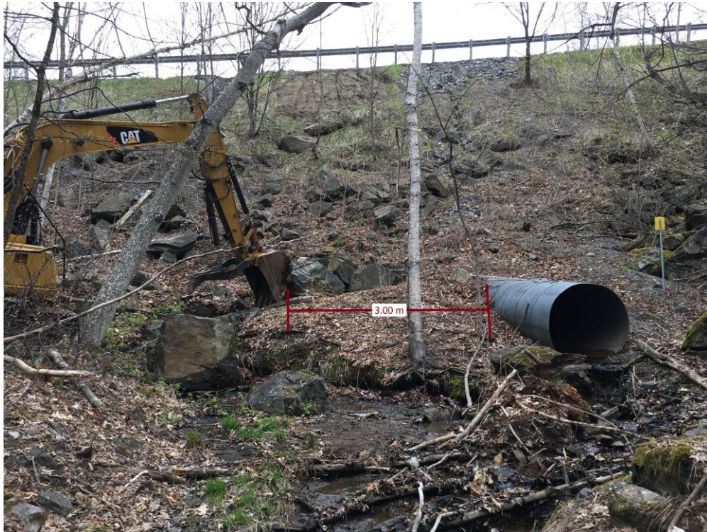
Photo 19: Test pit TP3 at the toe of west embankment slope facing west, outlet side
