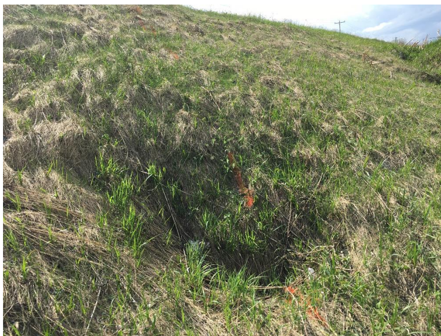
Photo 8. Sinkhole on west side slope at Culvert #2
