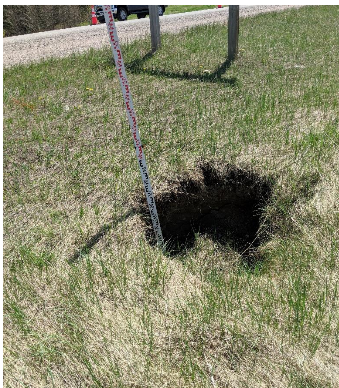
Photo 4. Sinkhole on west side slope at Culvert #1
