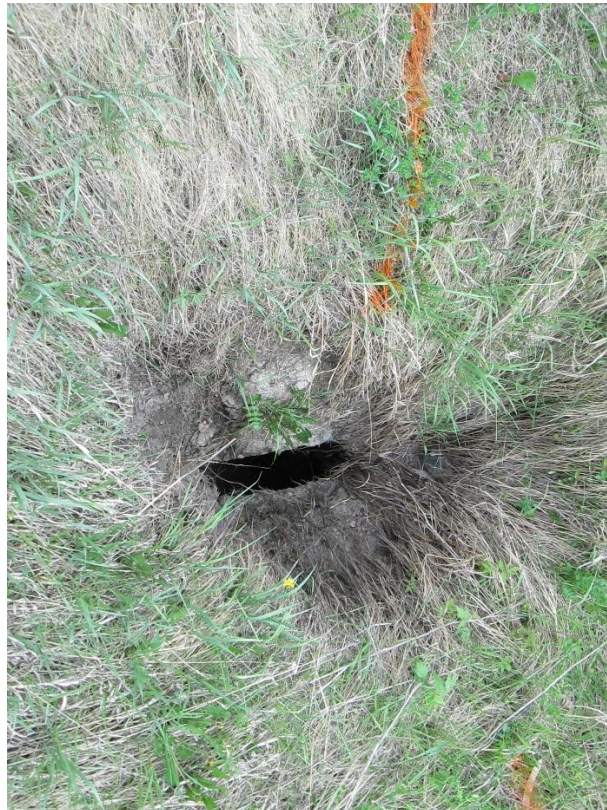
Photo 16. Sinkhole with separated culvert at west side slope at Culvert #3
