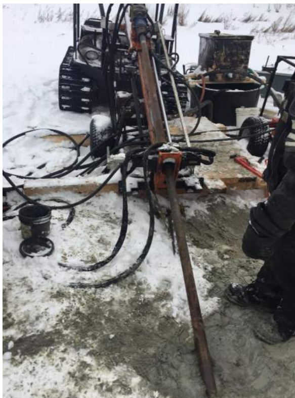
Photo 9. Drilling angled BH17-1
