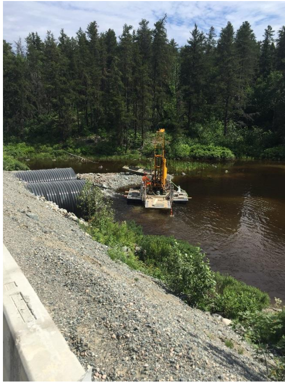
Photo 15. Borehole BH-1 drilling using a barge
