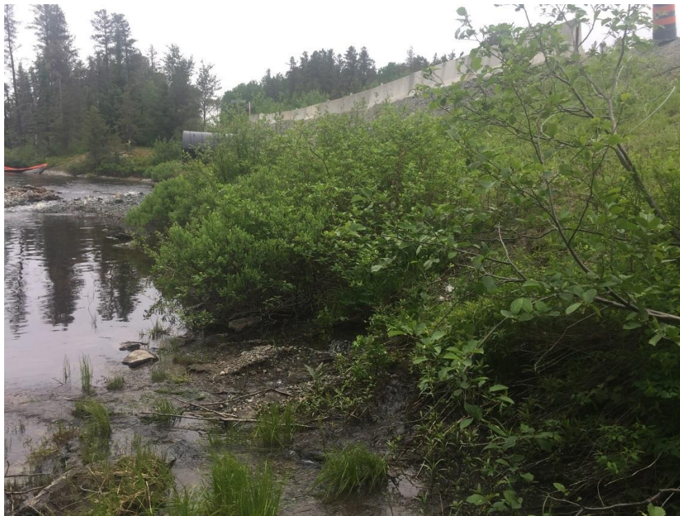
Photo 12. Water seepage through east(outlet) side of embankment north of existing culvert
