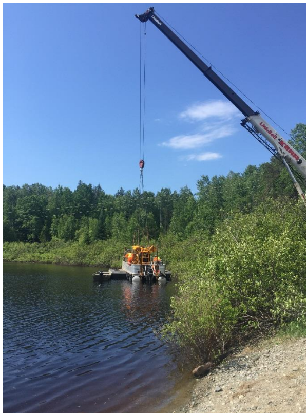
Photo 14. Crain lifting of barge and rig and placing them in water
