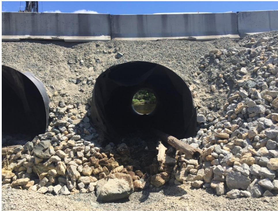
Photo 11. Temporary twin culvert, inlet side looking east
