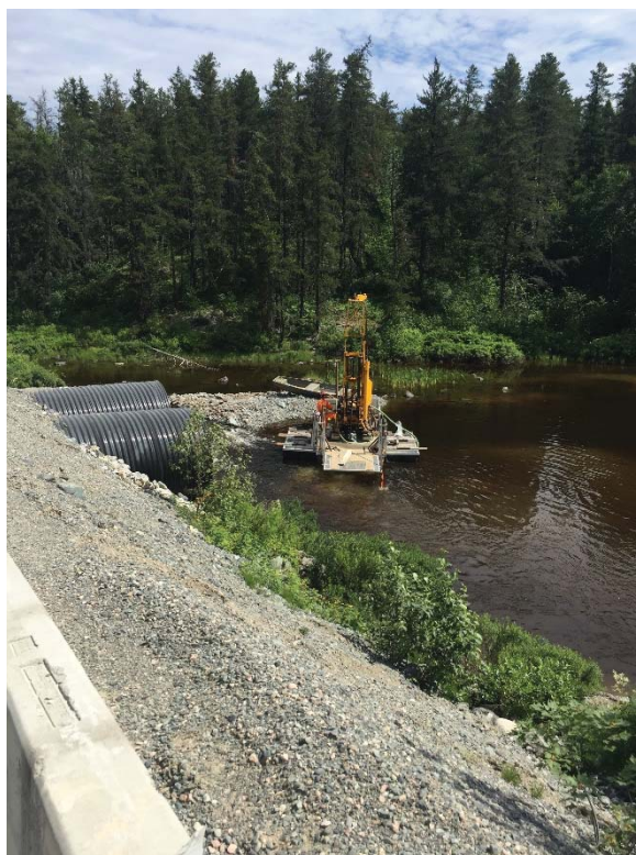
Photo 15. Borehole BH-1 drilling using a barge
