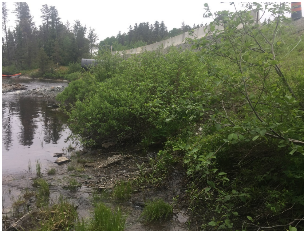
Photo 12. Water seepage through east(outlet) side of embankment north of existing culvert
