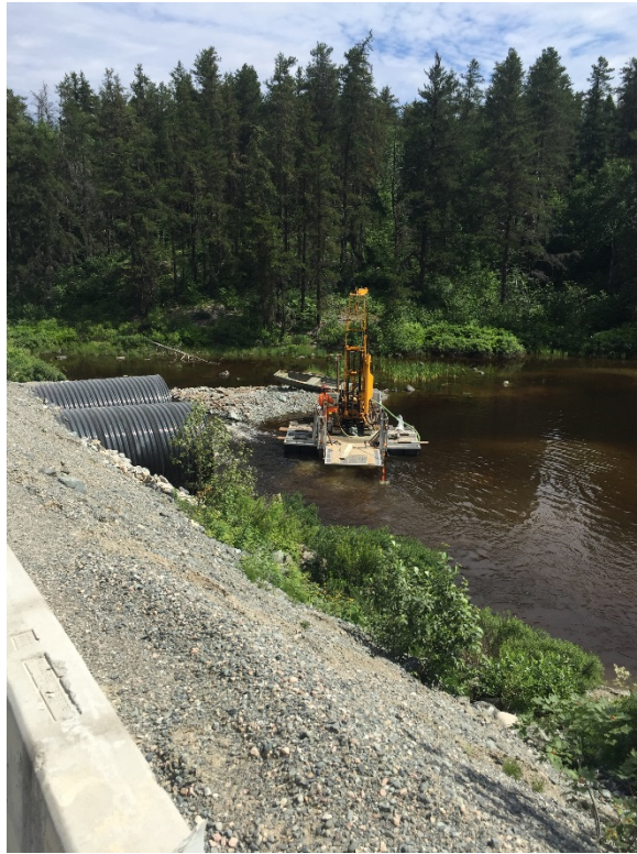
Photo 15. Borehole BH-1 drilling using a barge
