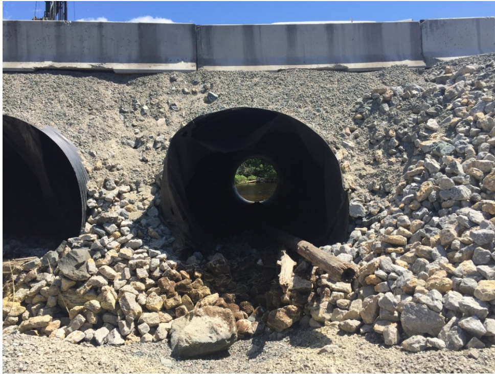
Photo 11. Temporary twin culvert, inlet side looking east
