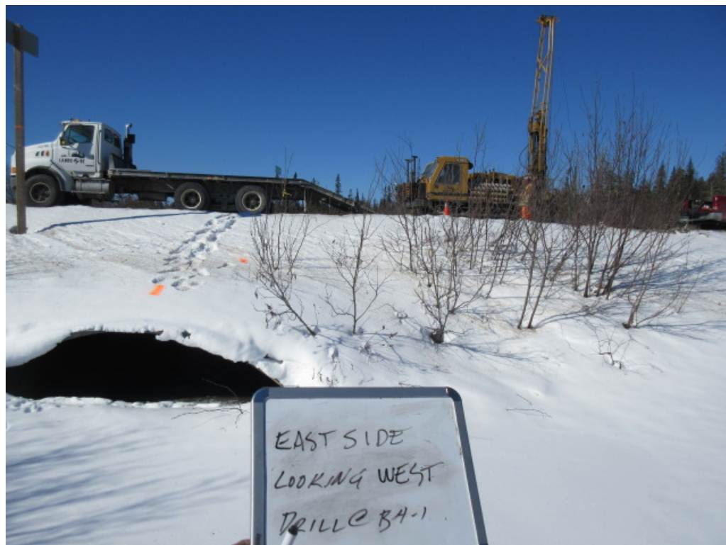
Photo 2. Drilling of BH1. Inlet of the existing culvert, facing West
