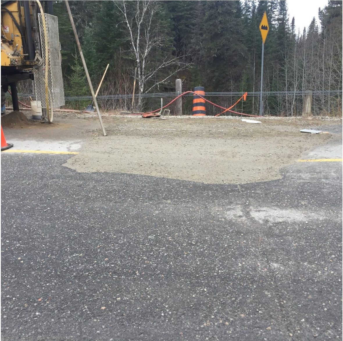
Photo 5. Temporarily Repaired Sinkhole on Western Side of Roadway (facing west) on November 8, 2016
