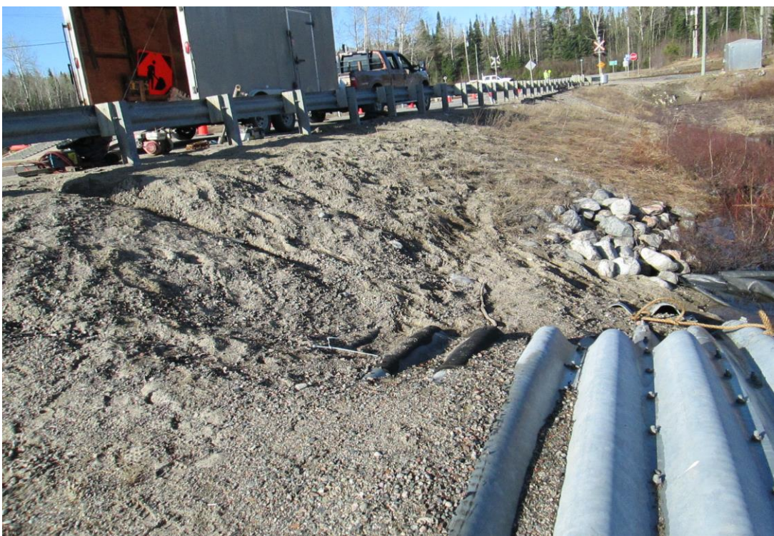
Photo 10. Washed away embankment slope on outlet side facing west
