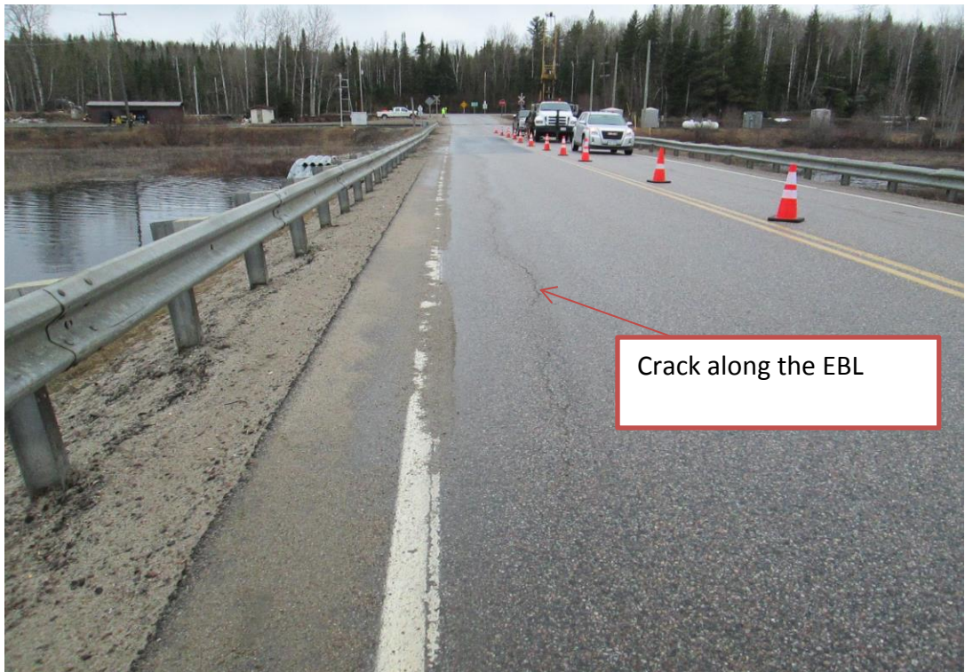
Photo 14. Typical crack on roadway along the EBL facing west
