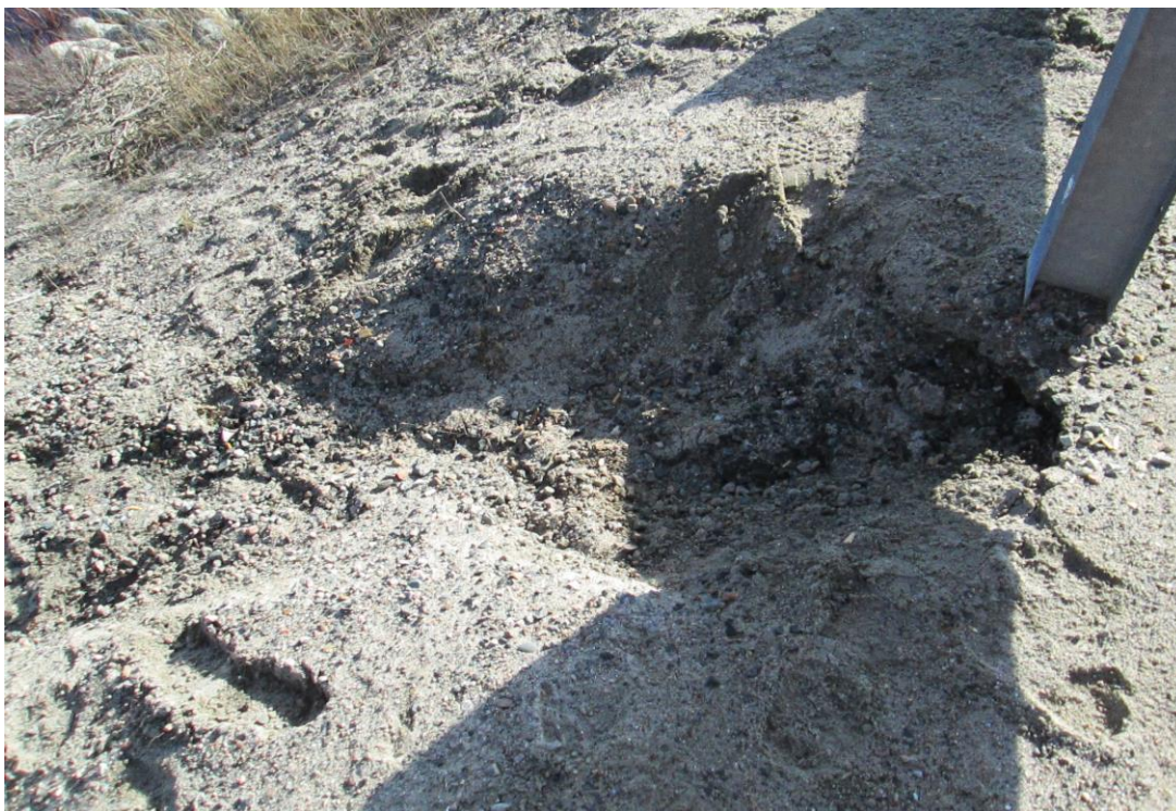
Photo 11. Washed away portion of embankment slope on outlet side
