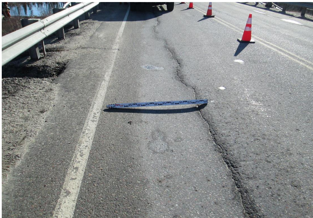
Photo 12. WBL roadway portion depressed on north-west half of embankment
