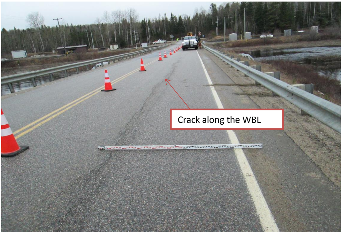
Photo 13. Typical crack on roadway along the WBL facing west
