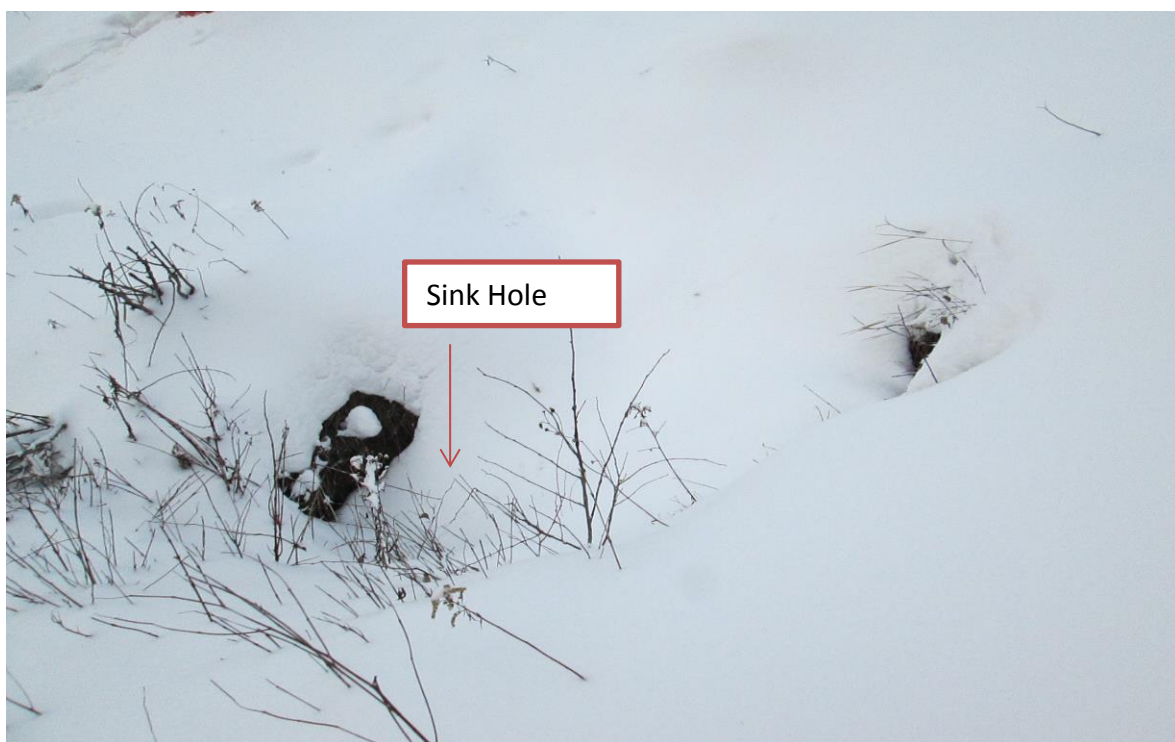
Photo 10. Sinkhole on south side (inlet) of embankment
