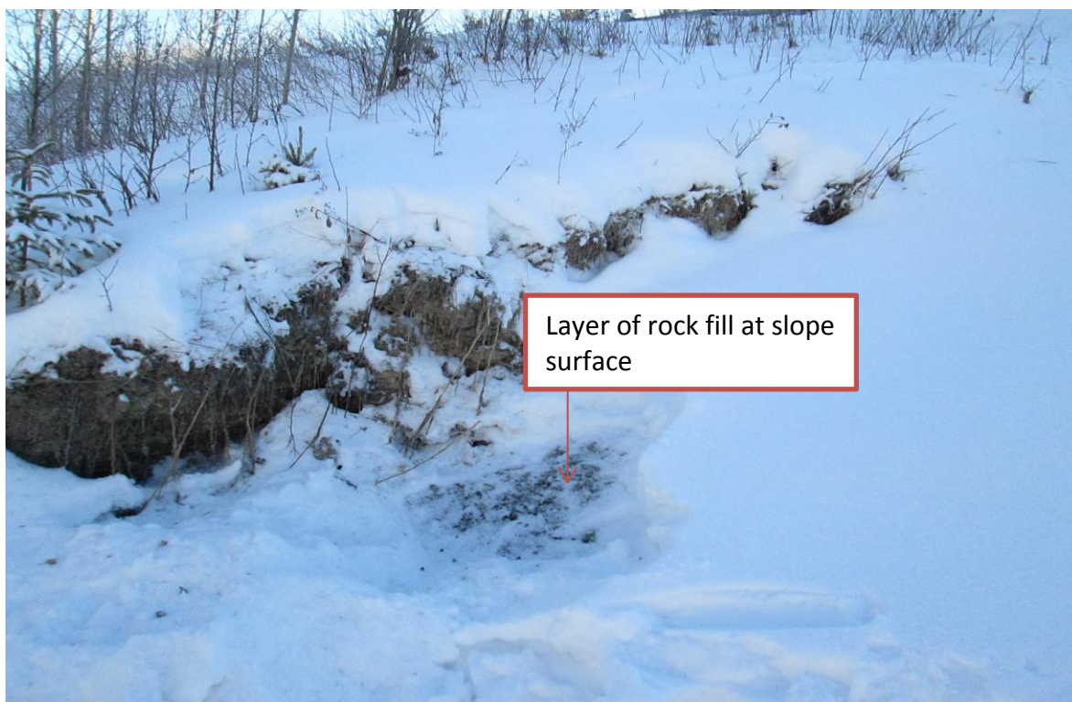
Photo 12. Depressed slope surface - north side (outlet) of embankment
