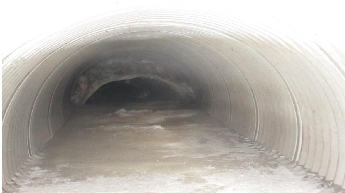
Photo 9. Blockage at culvert inlet side
