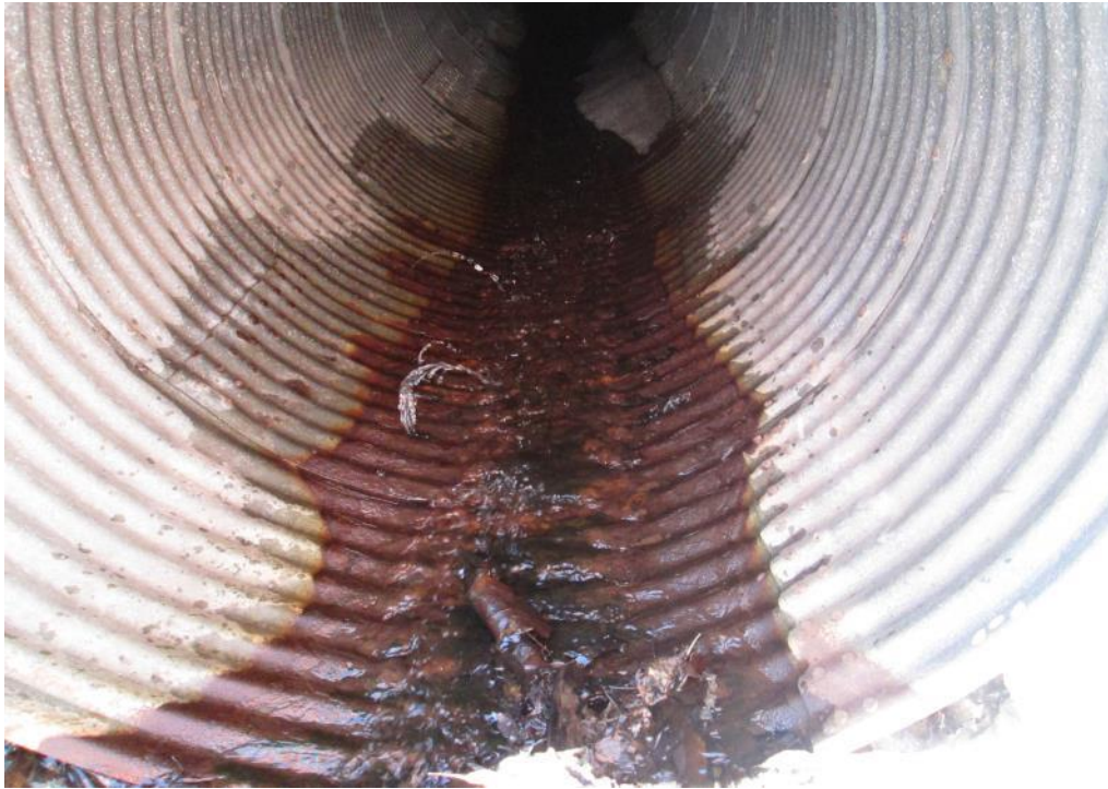
Photo 11: Deterioration of culvert at inlet
